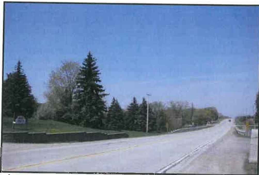
Plate 6: View north along Dixie Road approaching Creek near 12434 Dixie Rd (Ken Speirs Orchard Farm)
