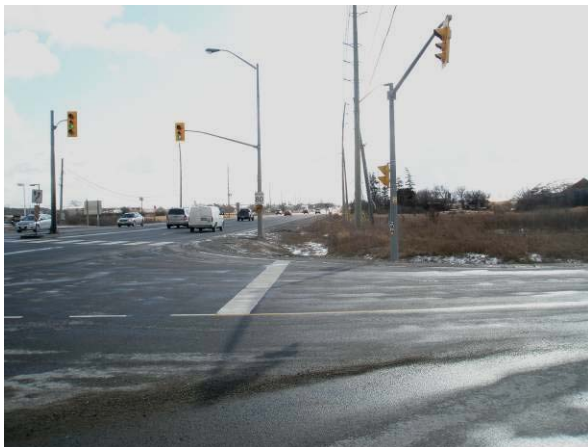
Plate 27: View south-southeast across Countryside Dr. at disturbed ROW at Highway 50 intersection.
