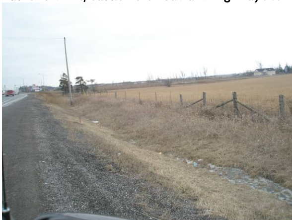
Plate 5: View south-southeast along Highway 50 at shoulder and wide ditch to fenceline.
