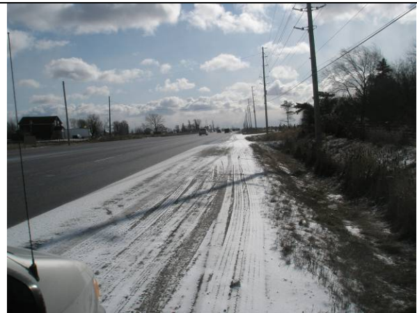
Plate 38: View south-southeast along Highway 50 at shoulder, ditch and sewer in disturbed ROW.
