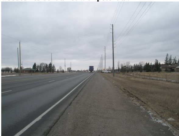
Plate 17: View north-northwest along Highway 50 at disturbed ROW to fenceline (at right).
