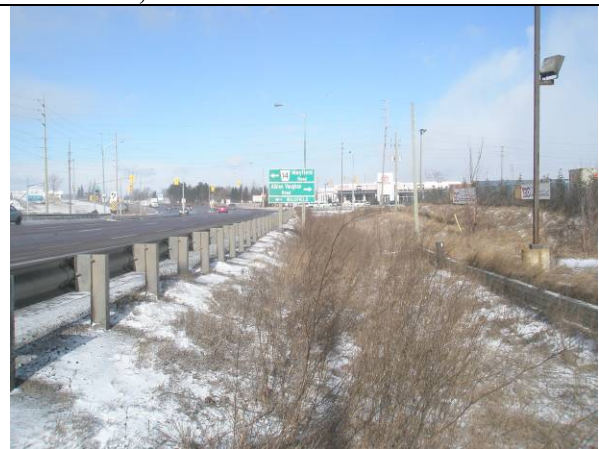
Plate 40: View north-northwest adjacent Highway 50 at severely disturbed lands at Mayfield Rd. intersection.
