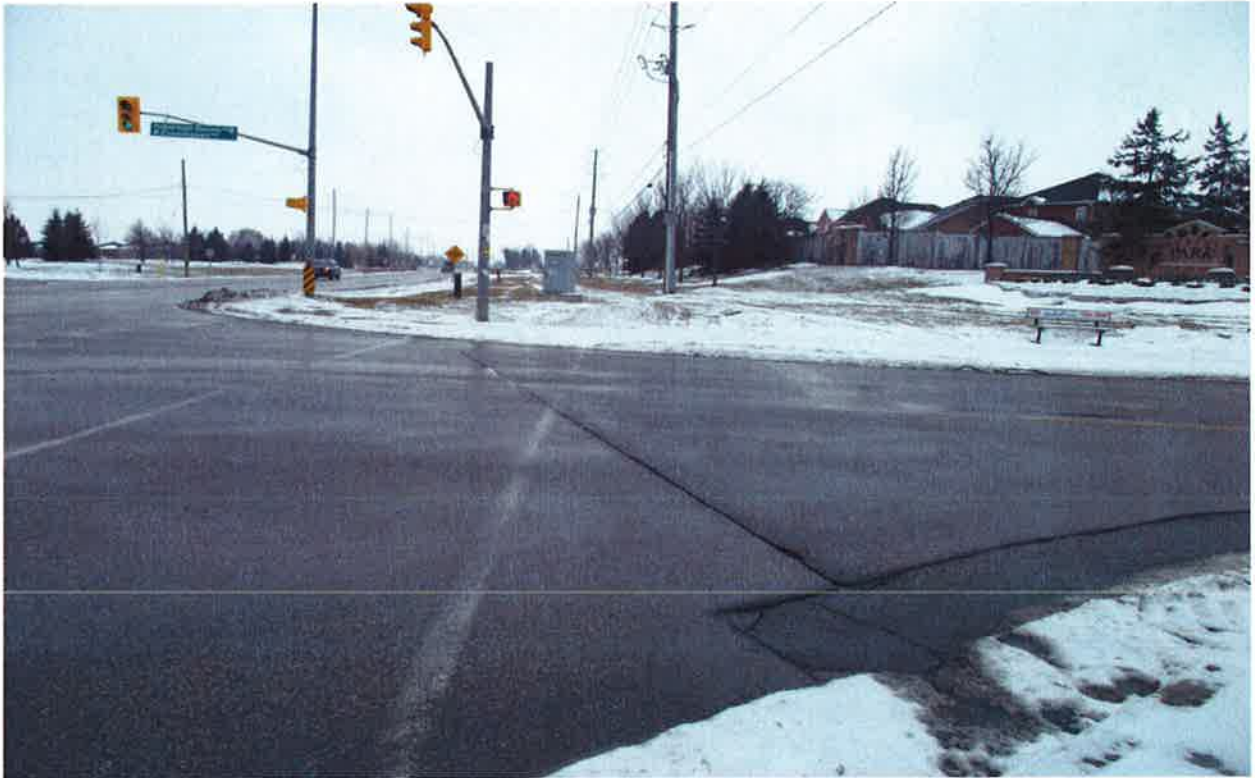
Mayfield Rd. and Robertson Davies Rd. Intersection\Section 2: Looking towards West
