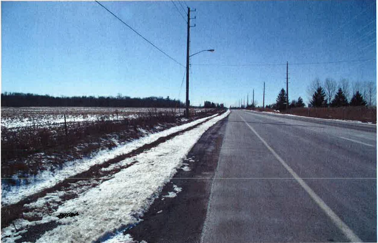
Mayfield Road\Section 1: Looking towards West
