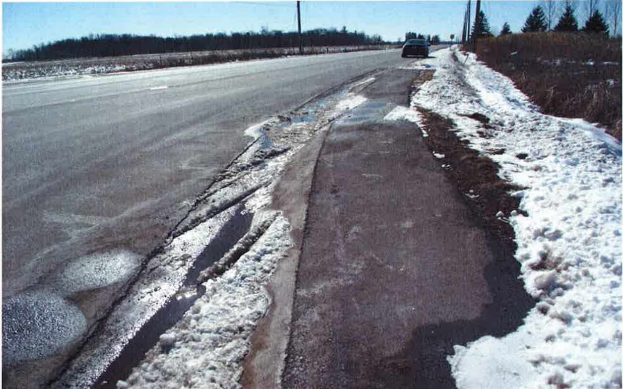
Mayfield Road\Section 1: Looking towards West
