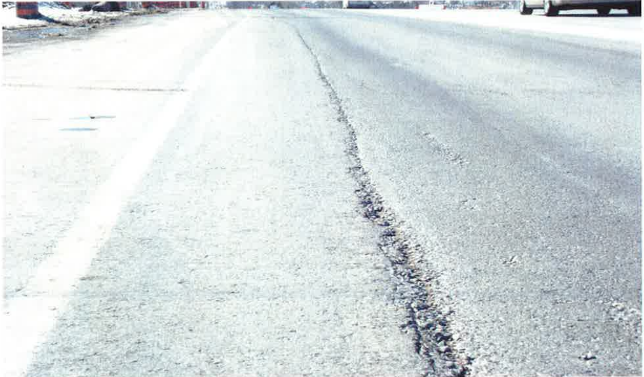
Mayfield Road\Section4: Looking towards West
