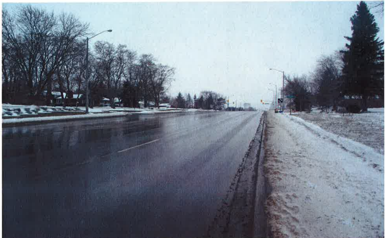
Mayfield Road\Section 3: Looking towards West
