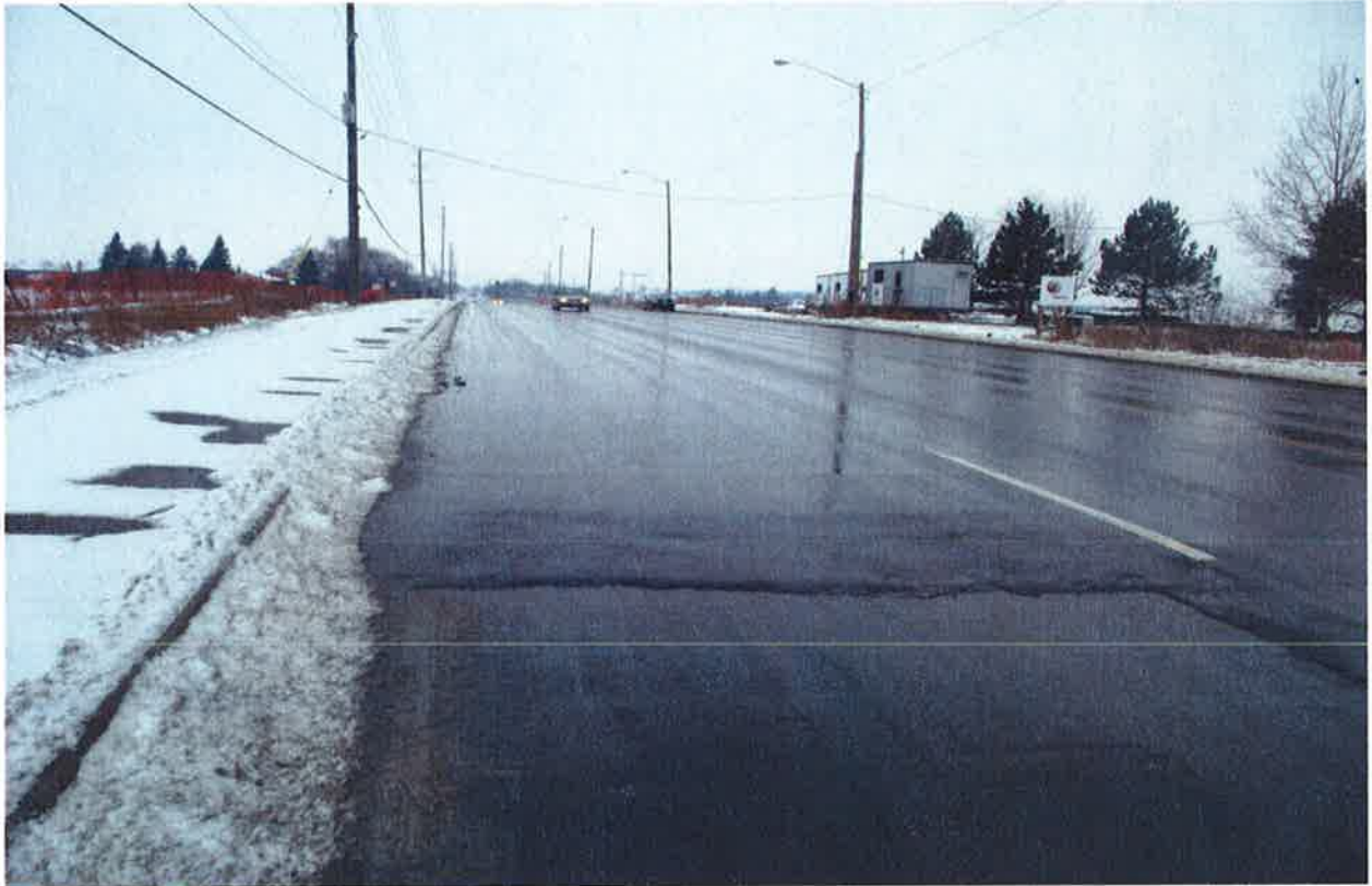
Mayfield Road\Section3: Looking towards West
