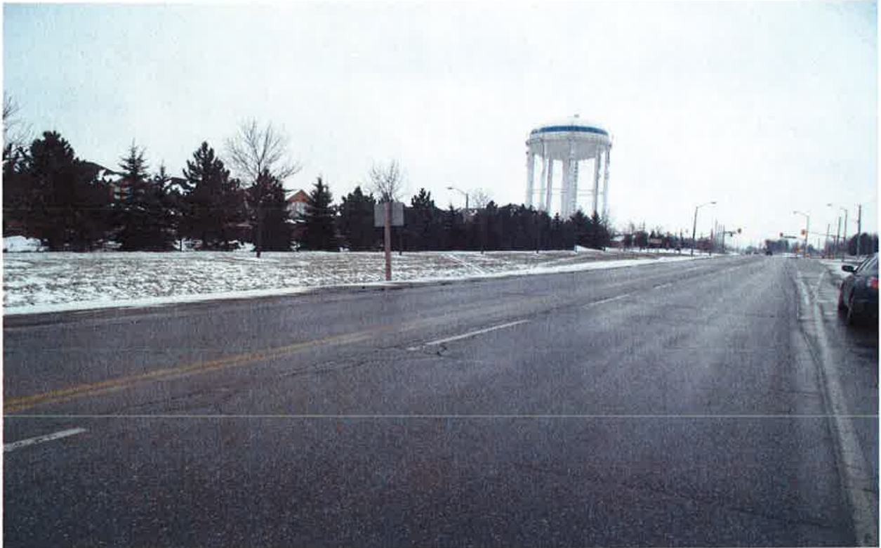
Mayfield Road\Section 2: Looking towards West, 400 m West of Hurontario Street
