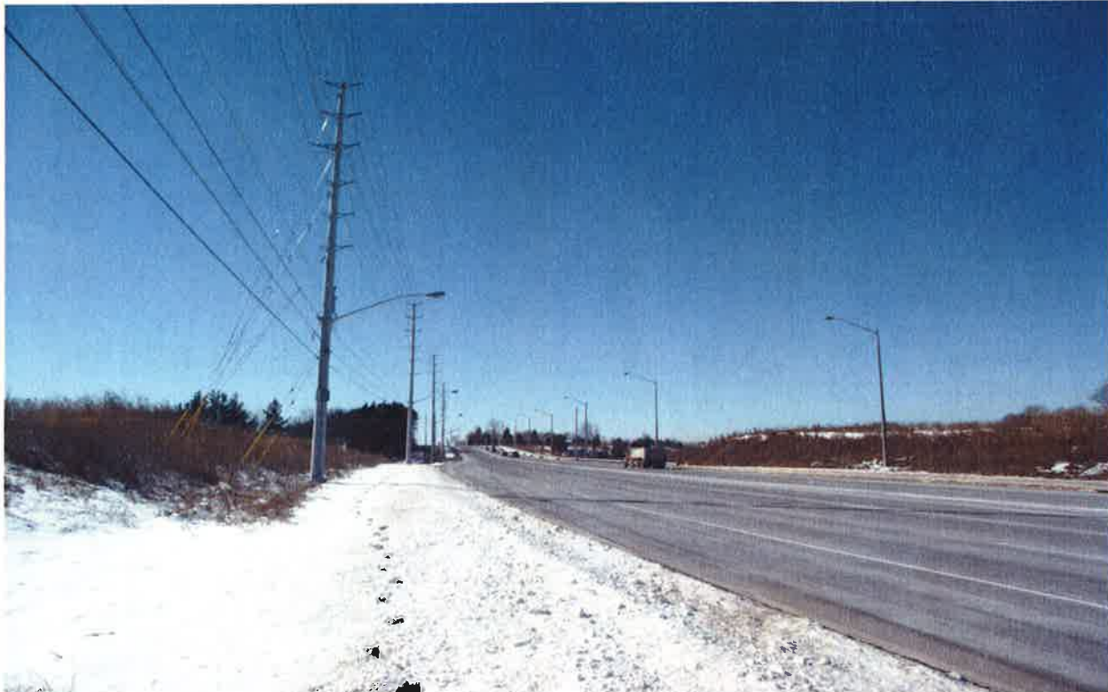
Mayfield Road\Section 5: Looking Towards West
