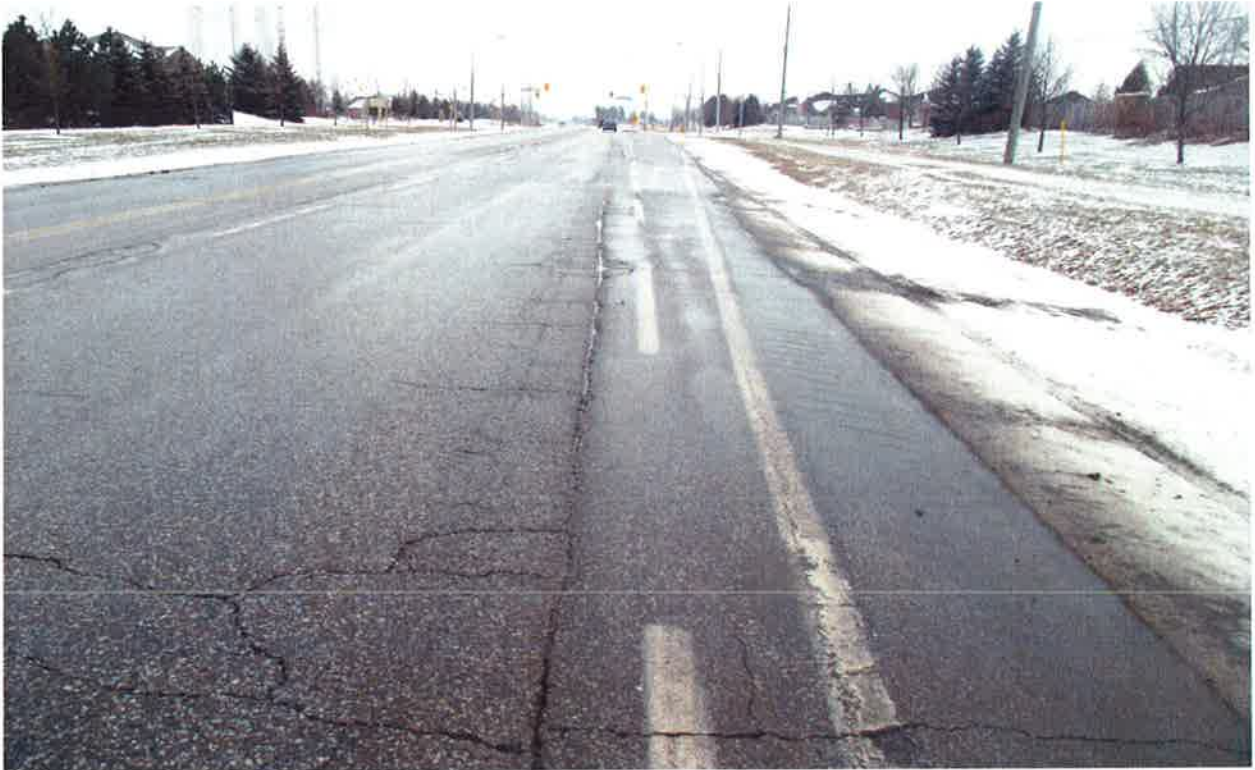
Mayfield Road\Section 2: Looking towards West
