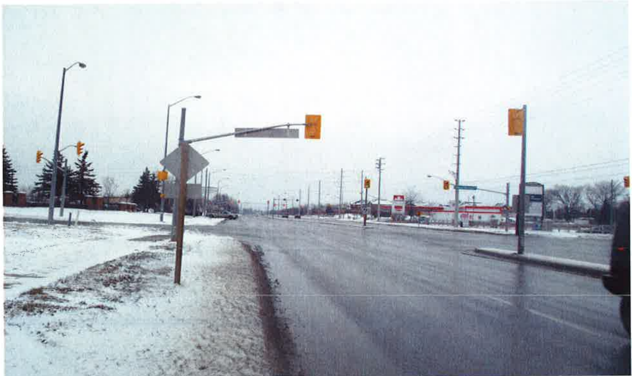
Mayfield Road\Section 3: Looking towards West, 200 m East of Hurontario St.\ Gas Station at the Northeast corner of Mayfield and Hurontario St. Intersection
