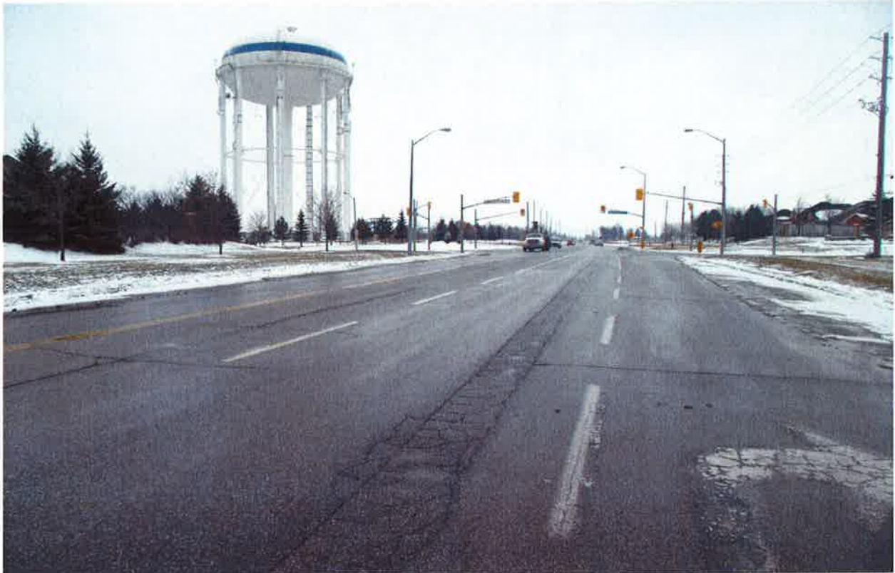
Mayfield Road\Section 2: Looking towards West
