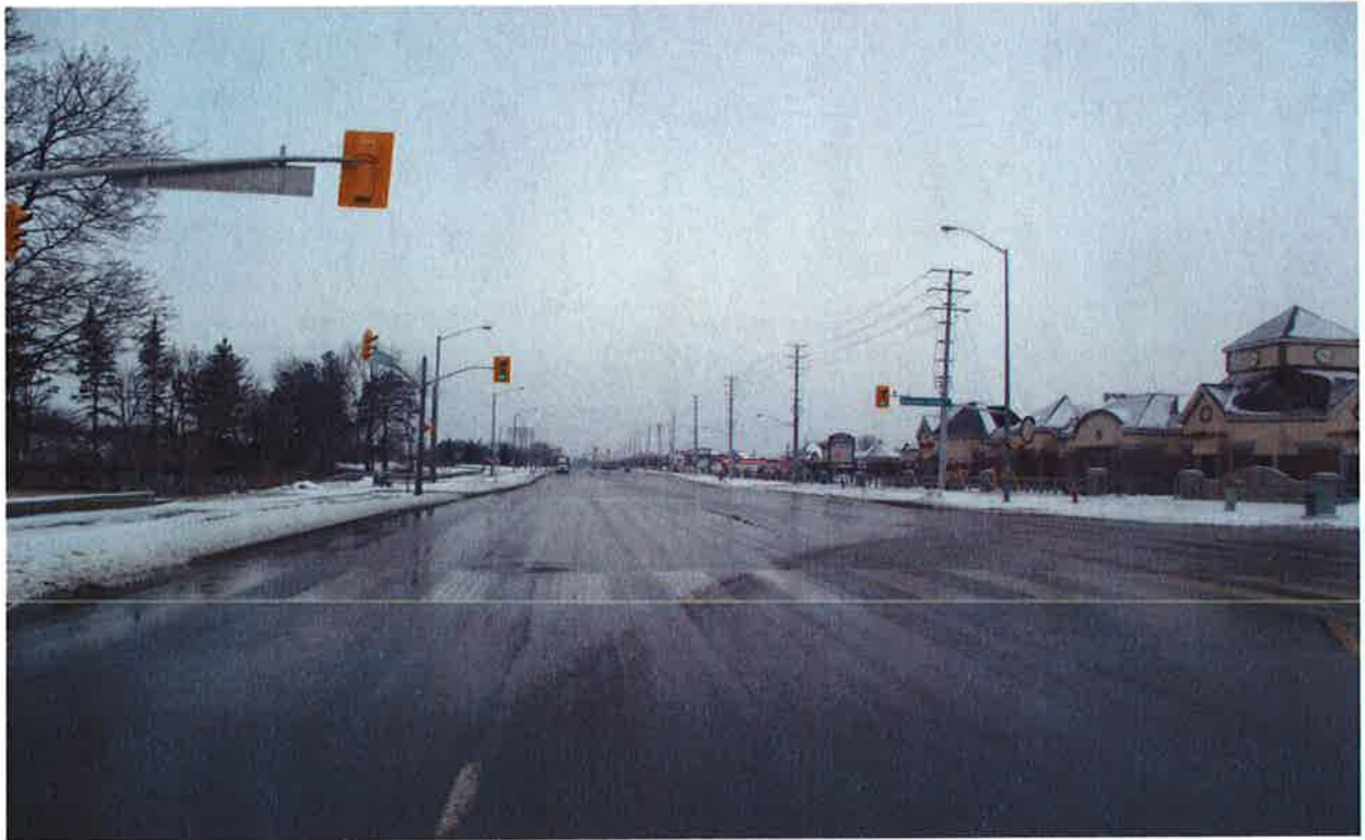
Mayfield Road\ Section 3: Looking towards West
