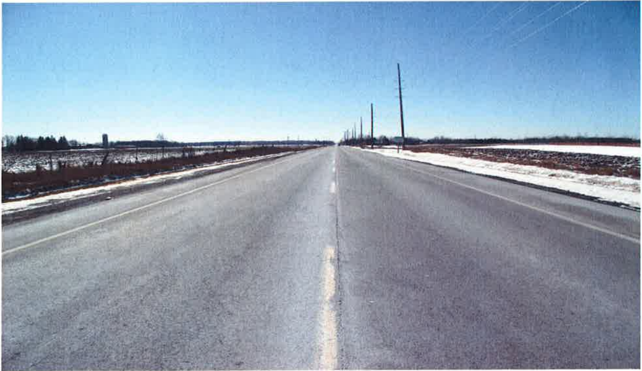
Mayfield Road\Section 1: Looking towards West
