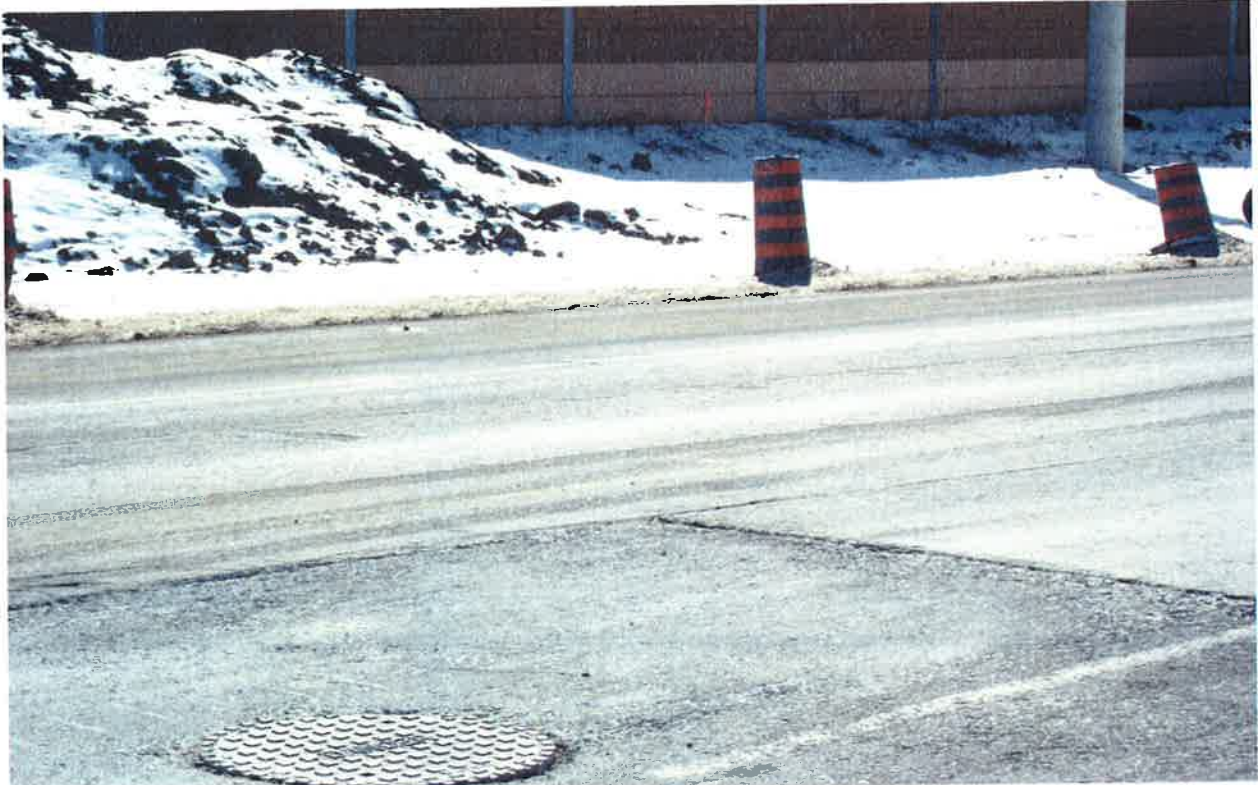
Mayfield Road\Section4\ Maintenance Treatment
