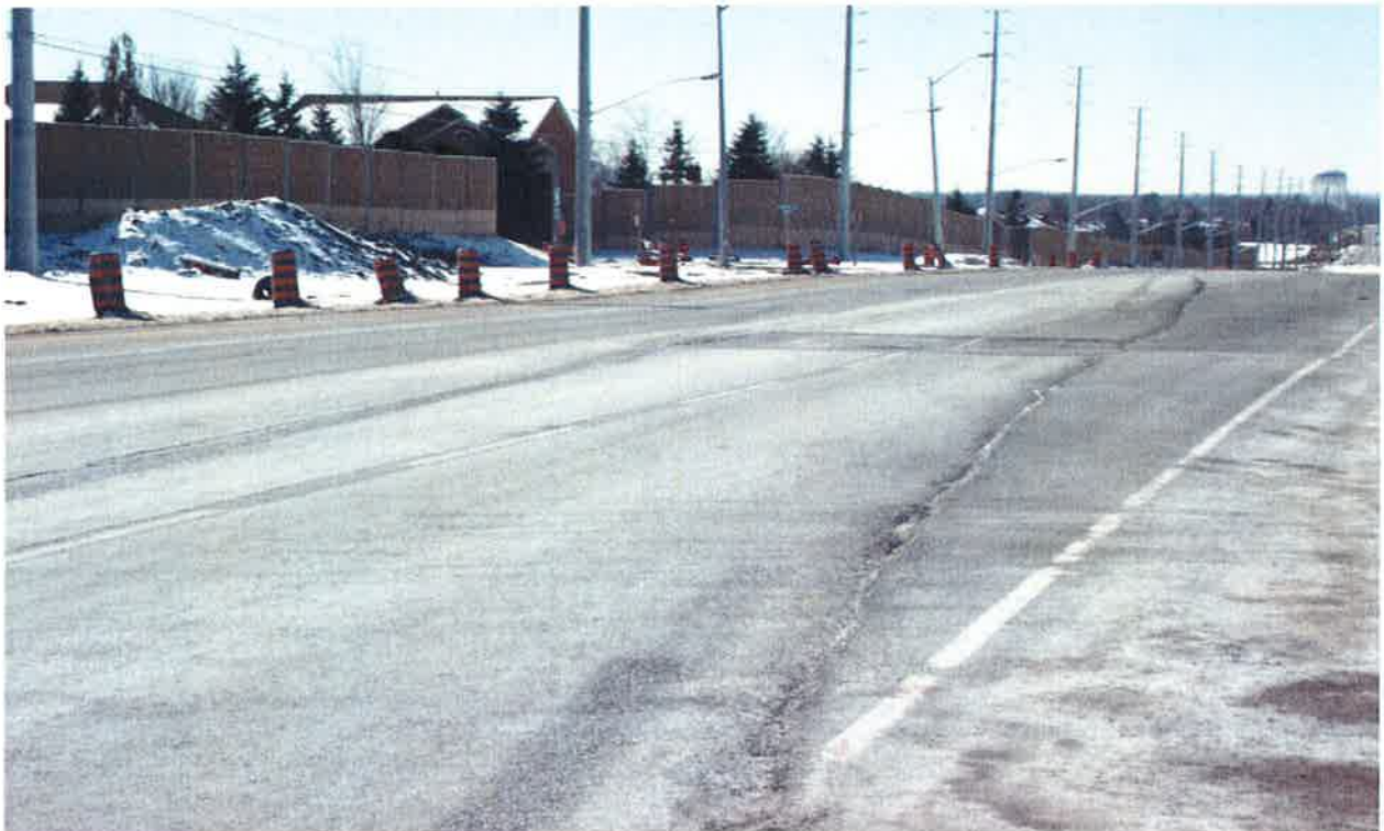
Mayfield Road\Section4: Looking towards West
