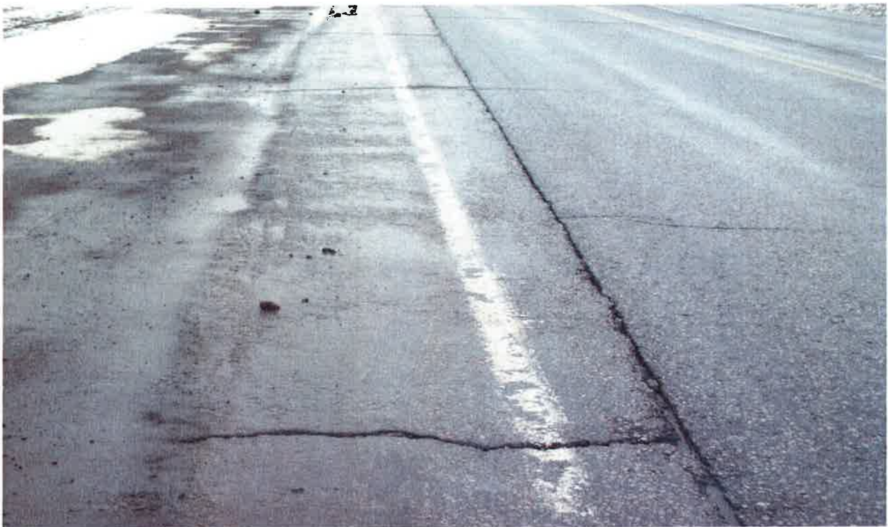
Mayfield Road\Section 2: Looking towards West, 500 m West of Hurontario Street
