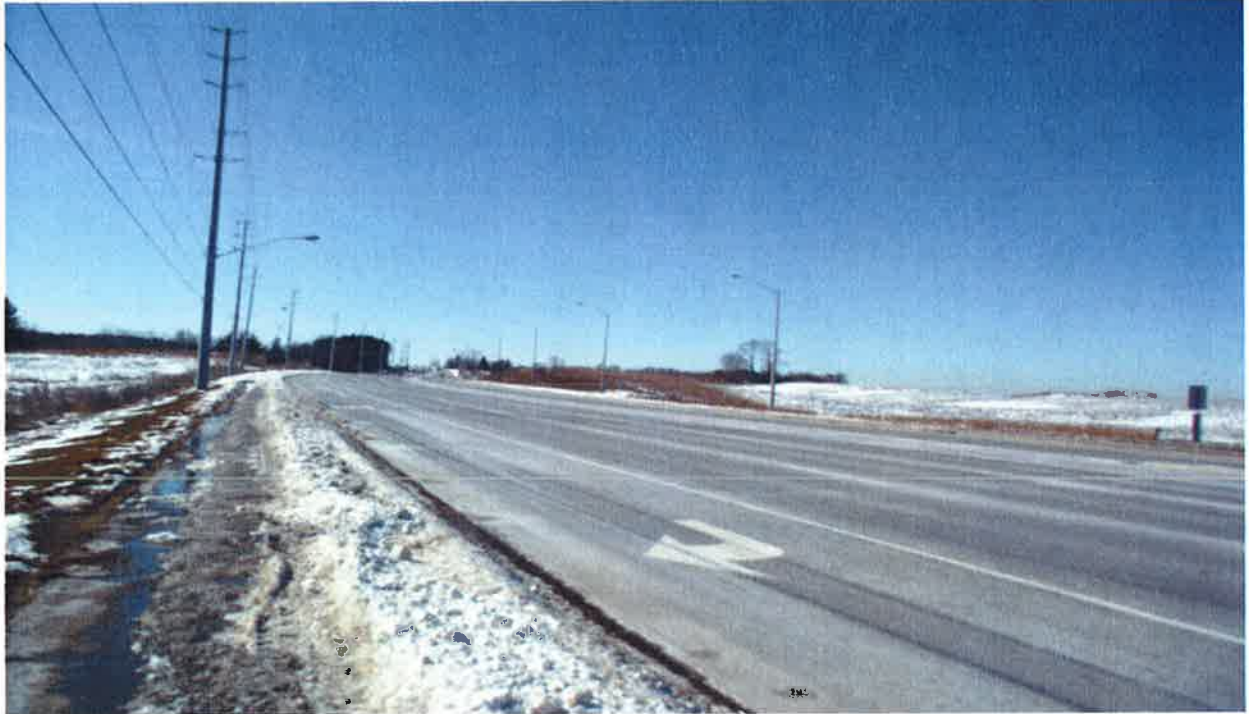
Mayfield Road\Section5: Looking Towards West
