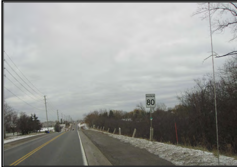
Figure 10: Replace marker post wire between Street 'A' and Healey Road
