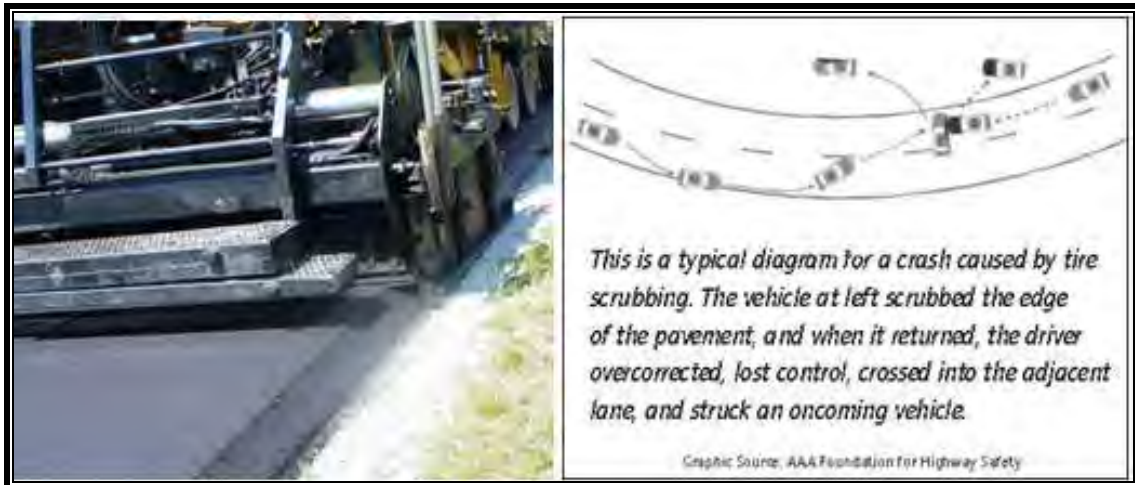
Figure 13: Safety Edge (Source - FHWA)
