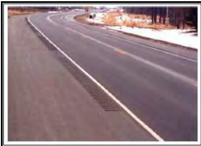
Figure 11: Shoulder Rumble Strip (Source - FHWA)
