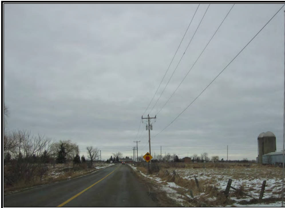
Figure 6: Advance Street Name Sign required on eastbound Old School Road
