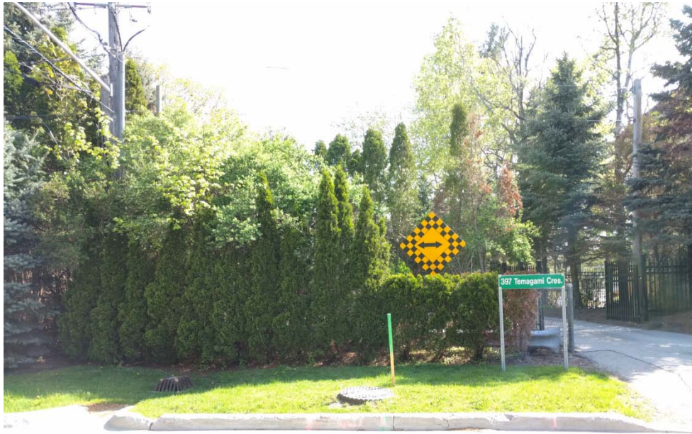
Plate 9: View of the Indian Road SPS from Temagami Crescent, looking north.
