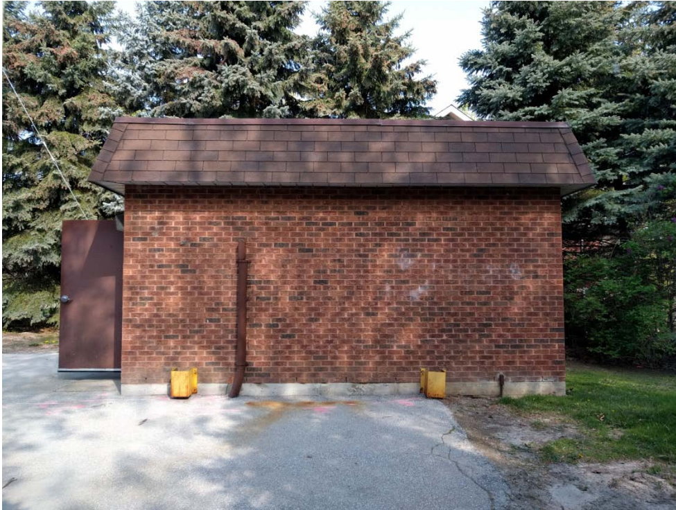
Plate 3: View of the Indian Road SPS diesel generation and control building, side elevation looking west.
