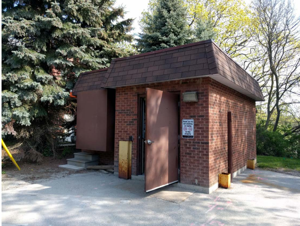
Plate 1: View of the Indian Road SPS diesel generation and control building, looking northwest.
