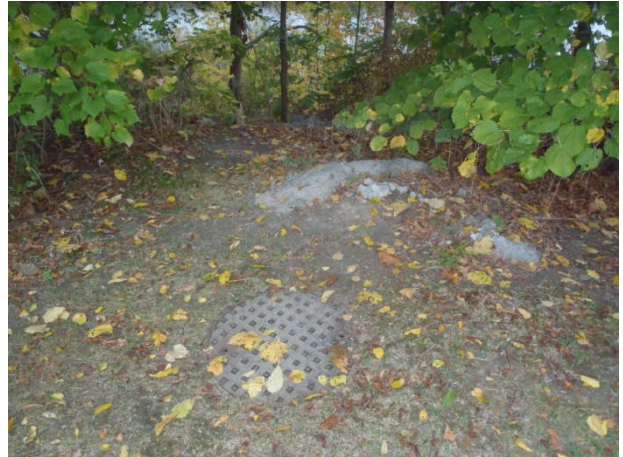
Plate 2: View northeast at previous disturbance at the Indian Road SPS study area.
