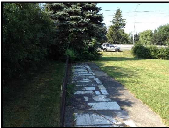
Image 7: Consolidated Monument (August 1, 2017; Facing Southwest)
