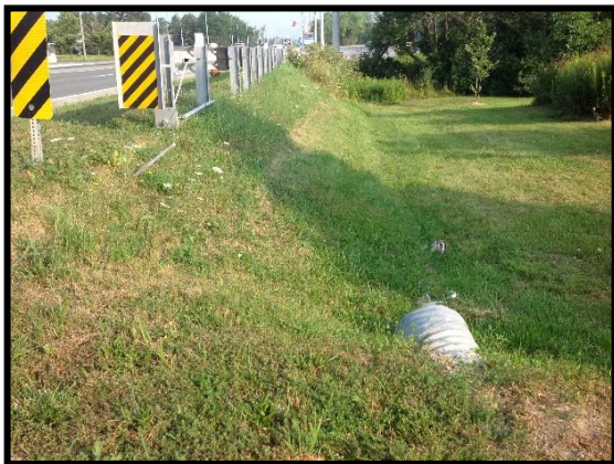
Image 3: Field Conditions (August 3, 2017; Facing Northwest)
