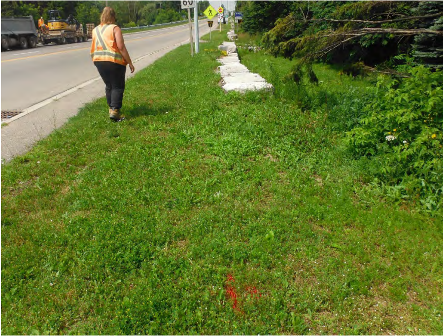
Image 7: Area of previous disturbance, subsurface utilities and slope to right of retaining wall, facing west-southwest
