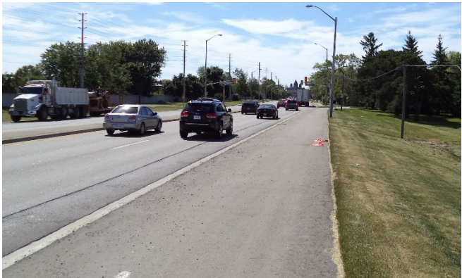
Multi-use path on the west side of Cawthra Road (North of Burnhamthorpe) – MTO Jurisdiction
