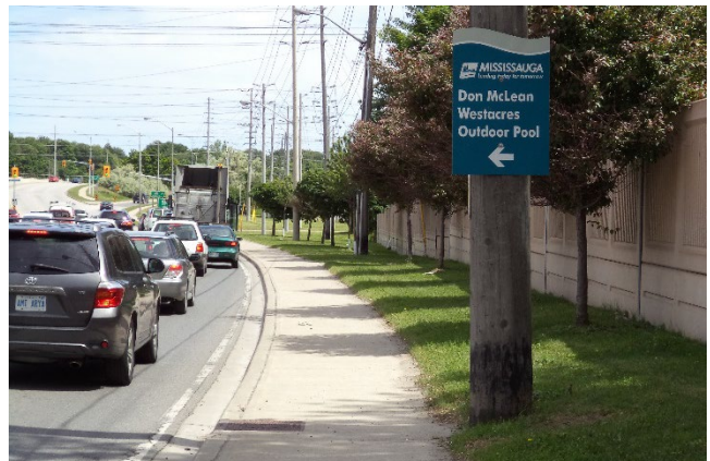
Curb-face Sidewalk (near Queensway)
