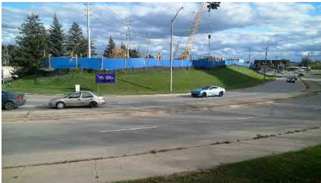
Photo 9. Limited areas of greenspace within Cawthra Right of Way (Oct 12, 2018).
