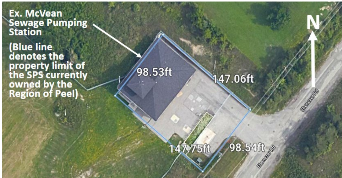
Figure 1-2: Existing McVean Sewage Pumping Station Property Limit
