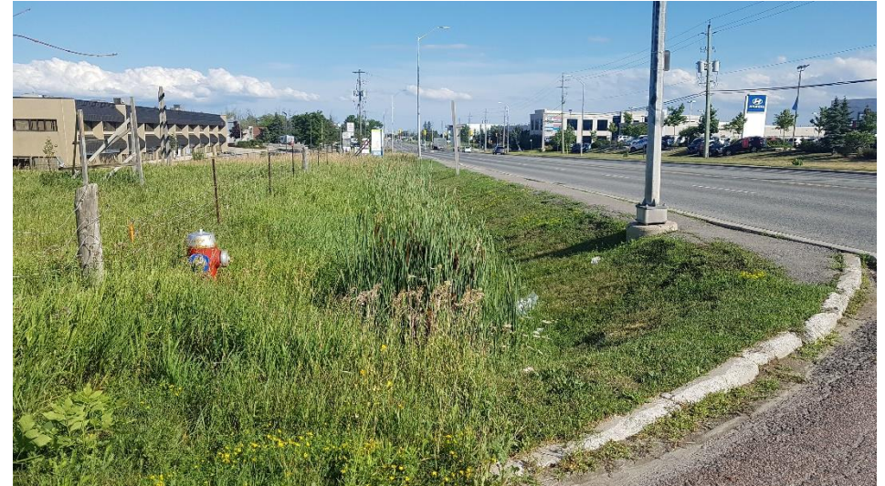
Image 10: View of disturbances associated with the asphalt roadway, concrete curbs, paved shoulder, buried utilities and ditching.
