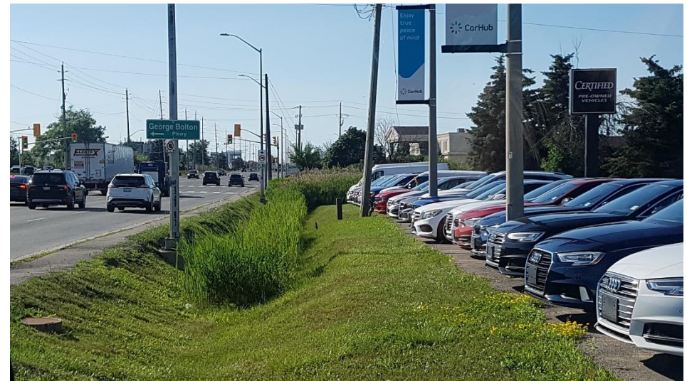
Image 8: View of disturbances associated with the asphalt roadway, concrete curb, paved shoulder, buried utilities and ditching.
