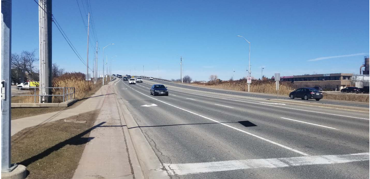
Photo 1: Highway 50 facing north at Healey Road intersection. The road raises several meters for a bridge structure over a CP Rail line below. Grass / vegetated ditches are visible on both sides of the road.
