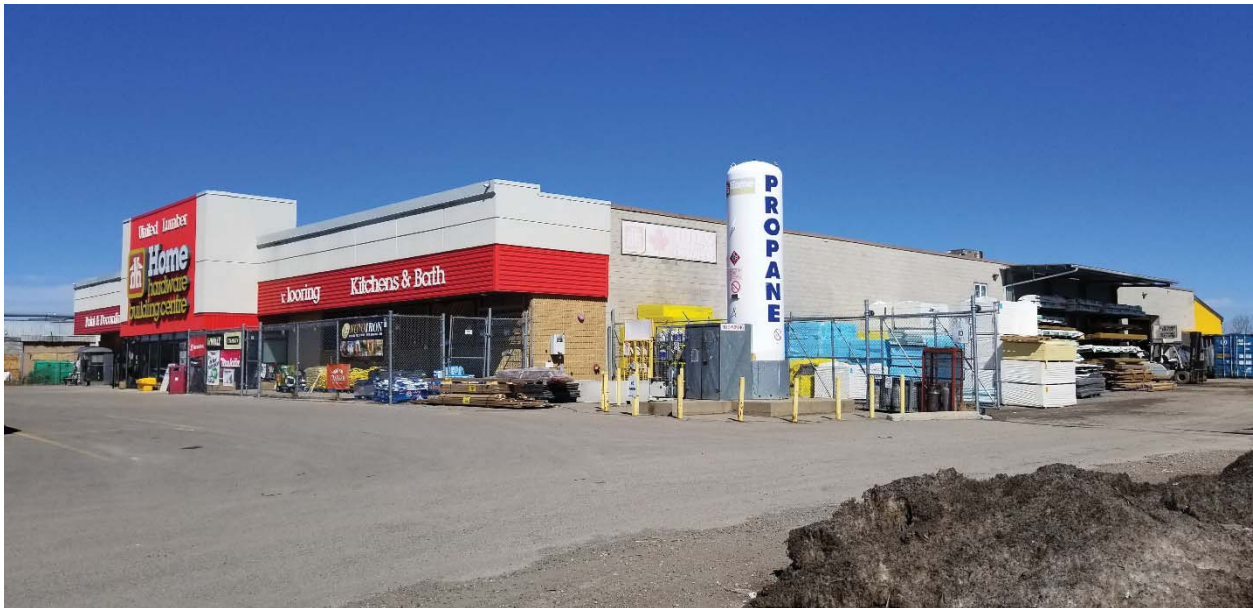
Photo 12: Home Hardware was located at 12833 Highway 50 at the north limit of the Site. A large propane storage tank was visible at the south west corner of the building, along with the storage of other unknown gas cylinders. Large stockpiles of treated lumber were visible at the rear of the store which neighbors the CP Rail corridor.
