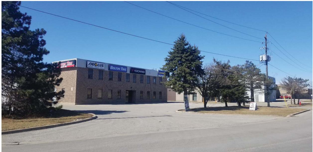
Photo 4: Bolton Tire Sales Inc auto service garage located at 770 Hardwick Road. Pole mounted hydro transformers are visible in the photo.
