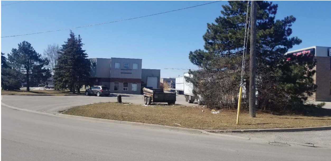
Photo 5: 780 Hardwick Road, historically used as a metal fabrication and manufacturing building and housed a wholesaler / distributor of industrial machinery and chemicals.
