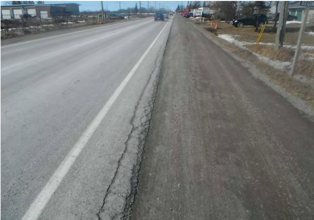
PHOTOGRAPH 4. Approximate Sta. 5+000, Airport Road, rural cross section, looking north.
