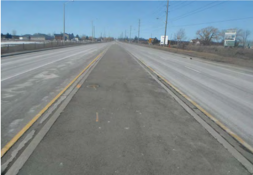
PHOTOGRAPH 1. Approximate Sta. 0+500, Airport Road, urban Cross Section, looking north.
