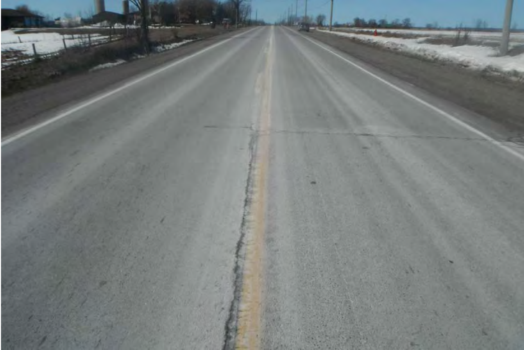
PHOTOGRAPH 3. Approximate Sta. 2+350, Airport Road, rural cross section, looking north.
