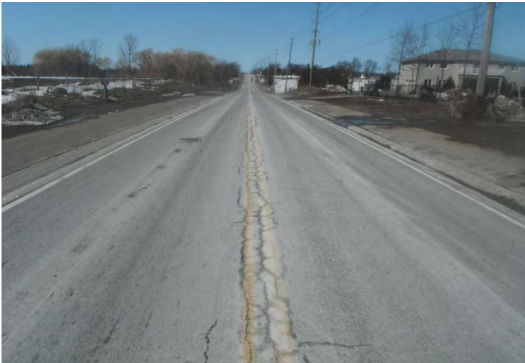
PHOTOGRAPH 2. Approximate Sta. 1+000, Airport Road, urban cross section, looking north.
