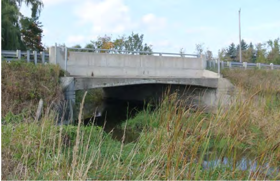
Plate 5: Detail of the east elevation, looking northwest.
