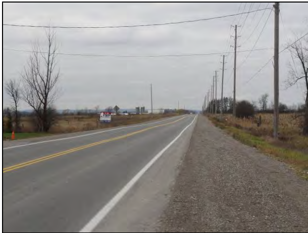
Plate 1: Looking north along Airport Road. Note the wide gravel shoulders.
