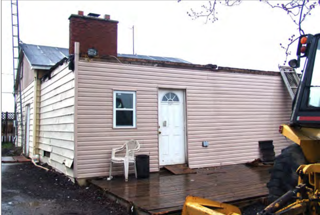
East facade (flat roofed addition), 2011
