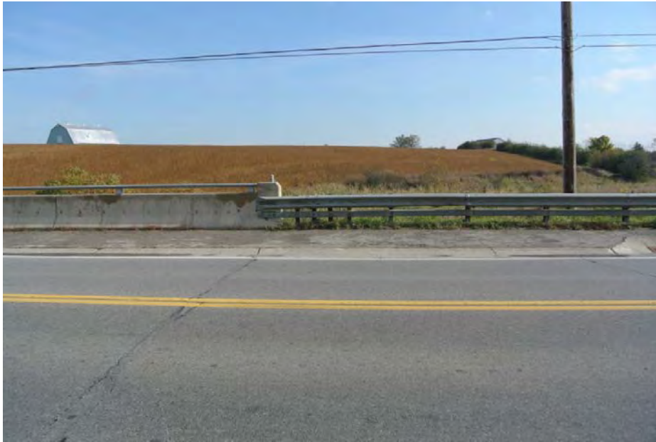
Plate 9: Detail of metal barrier system and concrete railing system located at the southeast corner of the bridge.
