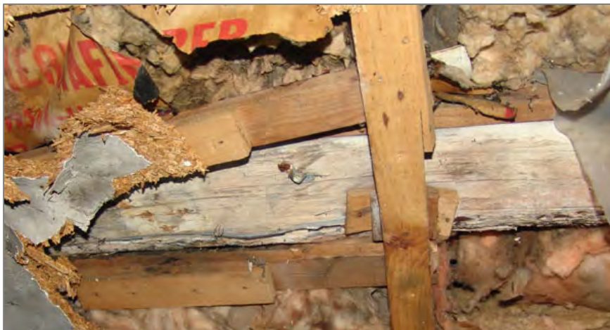
Below: Second floor, south room, showing timber/log with bark in ceiling/roof structure
