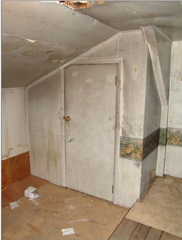
Above: Second floor, south room, southeast corner
