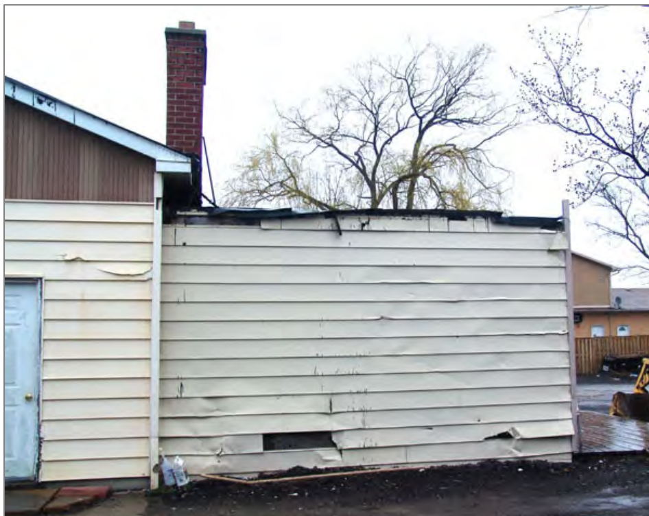
Below: South facade of east addition, 2011
