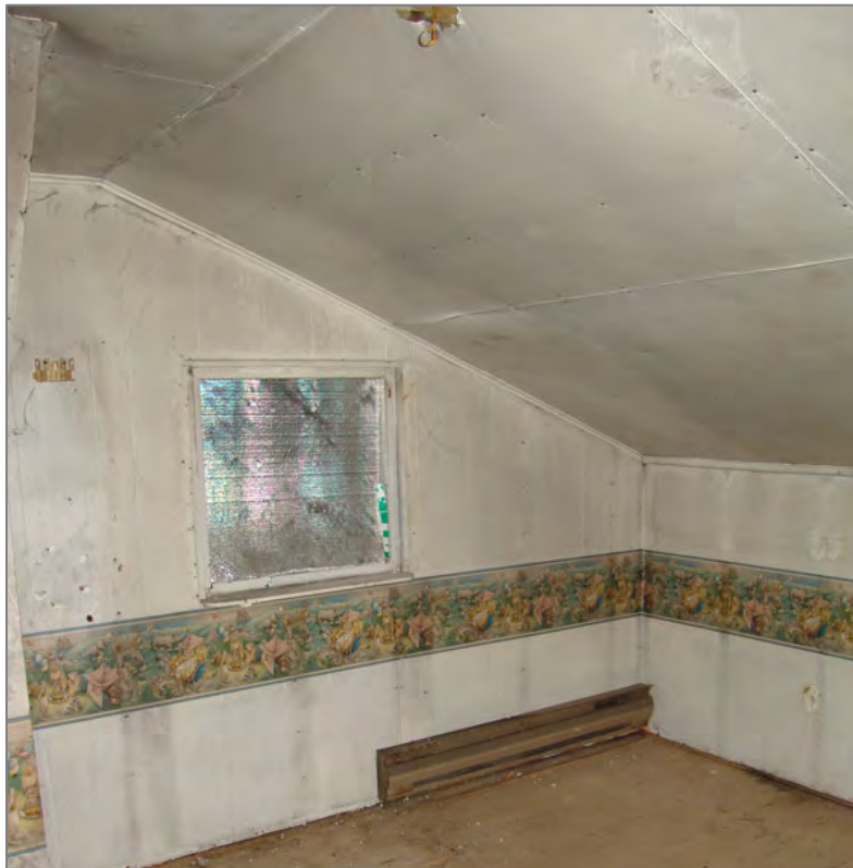
Below: Second floor, south room, south wall (L), west wall (R)
