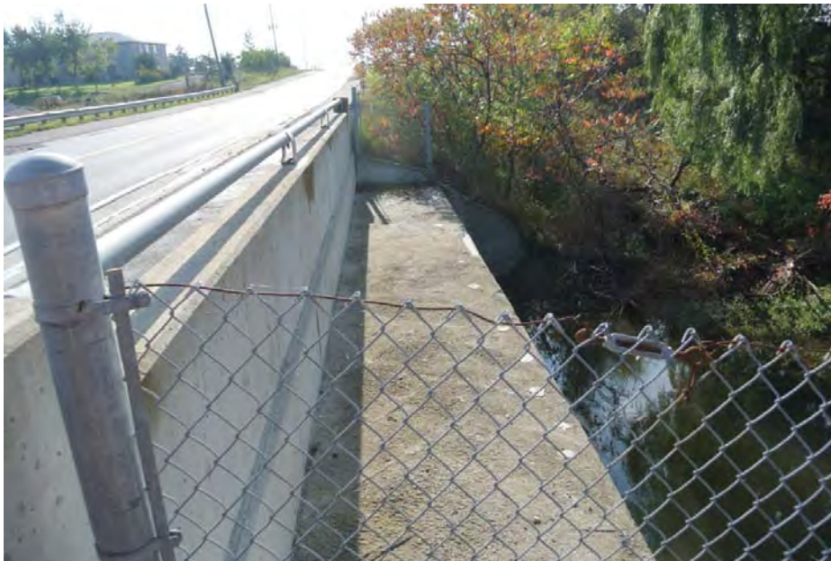
Plate 4: Oblique view of west elevation, looking south.
