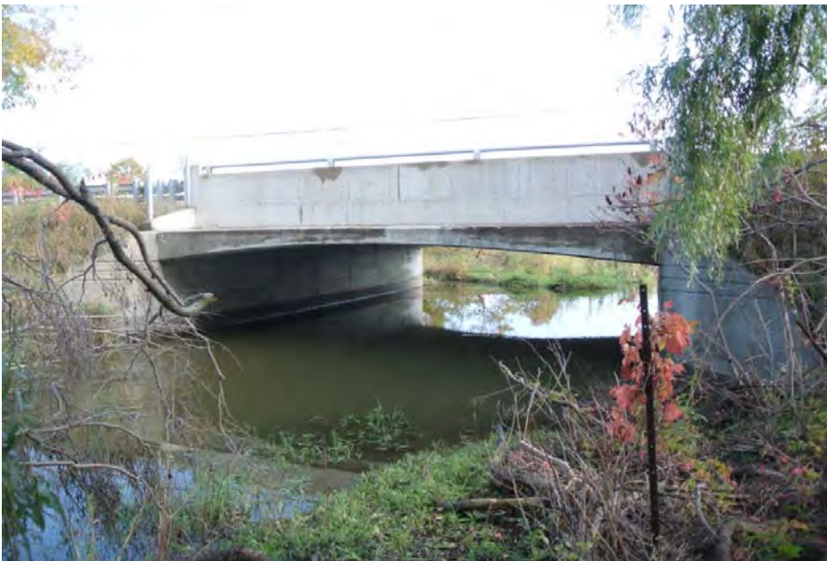
Plate 2: West elevation of the bridge, looking northeast.
