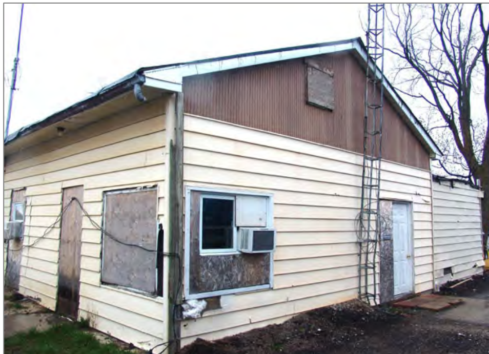
Below: West facade (L); and south facade, 2011
