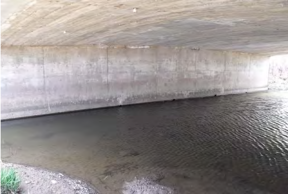
Plate 15: Detail of the bridge soffit and south abutment, looking southwest.
