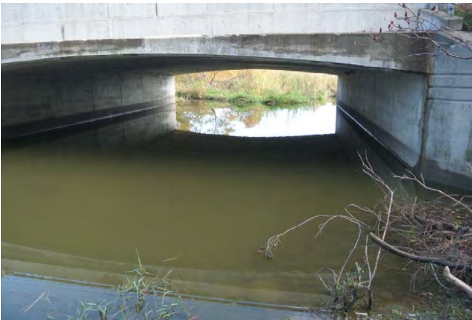
Plate 12: View underneath the bridge, looking east.
