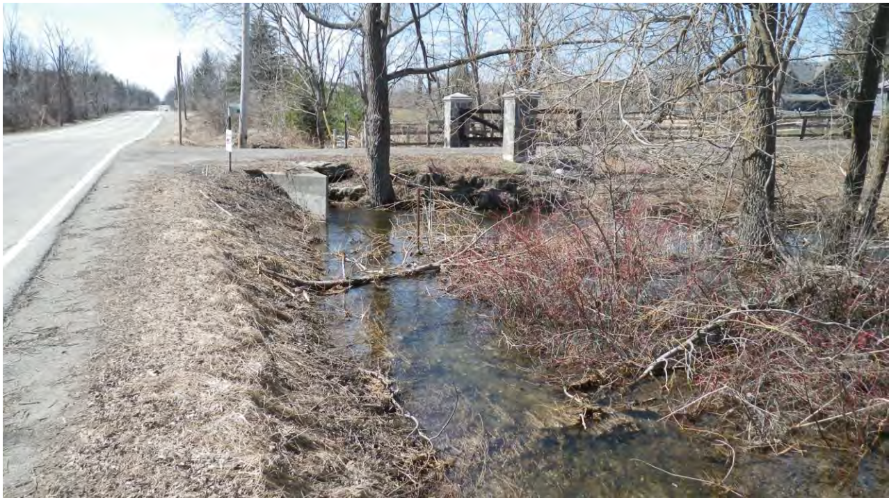
Photo 22: View looking downstream of roadside ditch which drains into culvert inlet.
