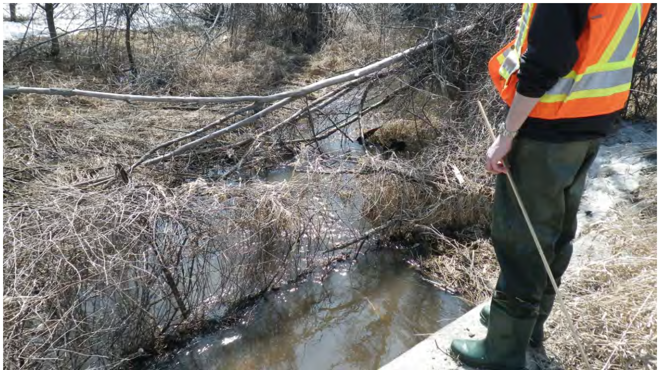
Photo 20: View looking downstream from culvert outlet.
