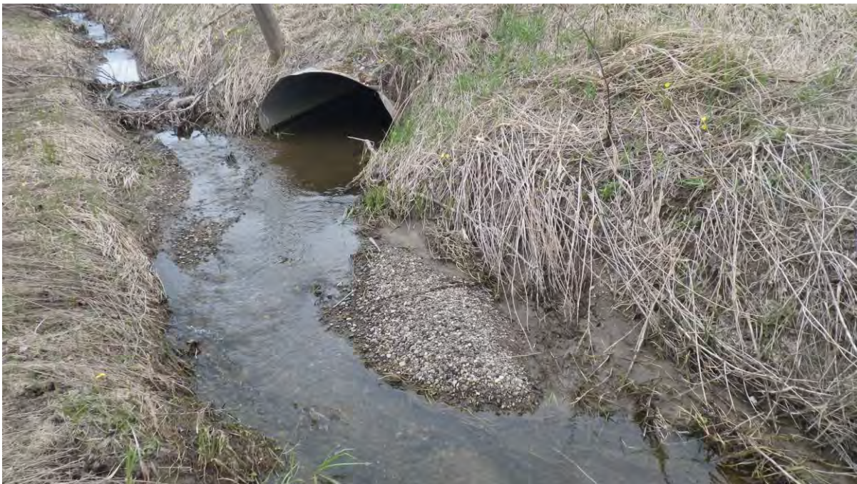
Photo 12: View looking upstream towards culvert outlet.
