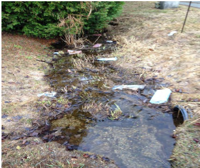
Photo 10: View looking downstream of culvert.
