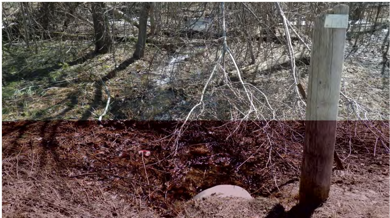
Photo 18: View looking upstream of culvert inlet.
