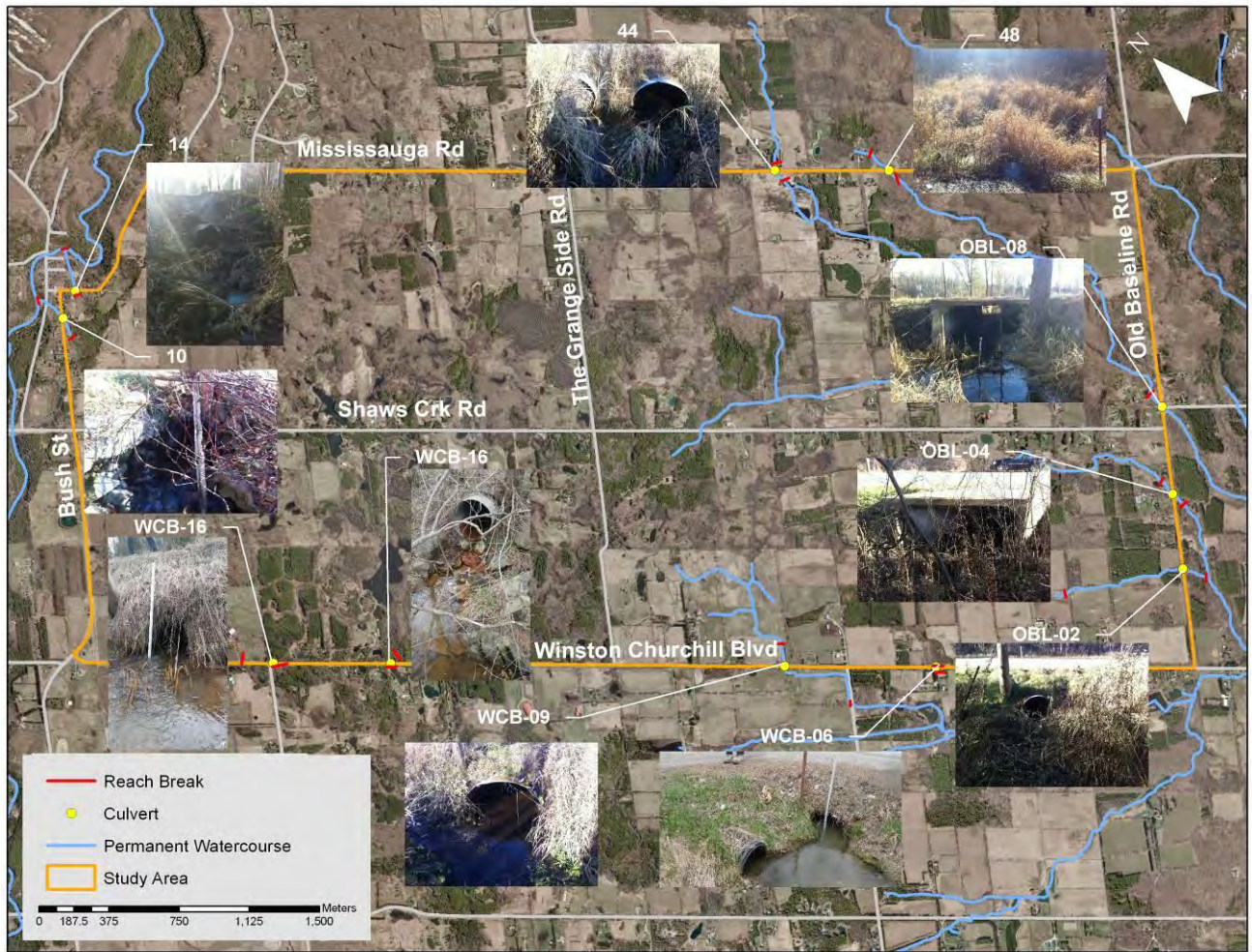
Figure 5.1: Culvert structures photographed at each crossing location.
