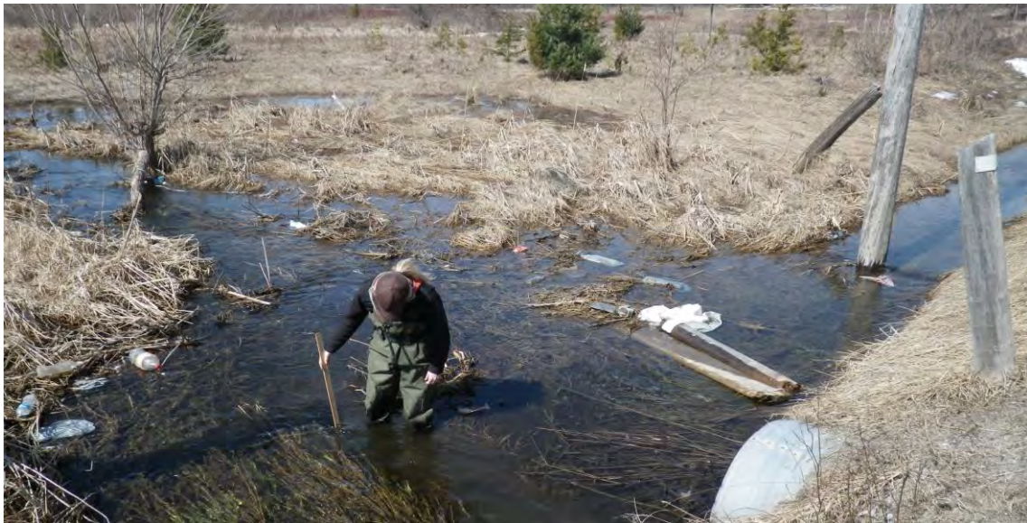
Photo 2: View looking downstream of culvert outlet towards marshy area.
