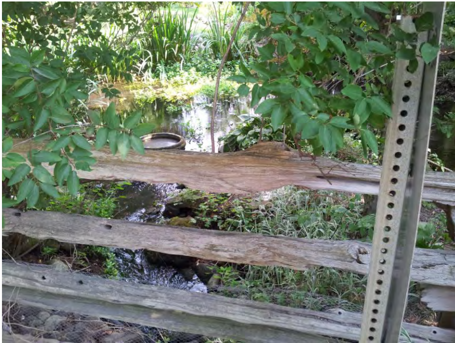
Photo 5: View looking upstream of culvert crossing at online pond.
