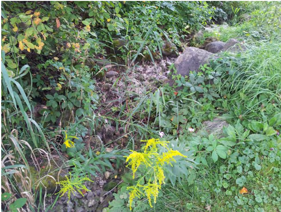
Photo 7: View looking upstream of culvert crossing at dry, steep, artificial channel.
