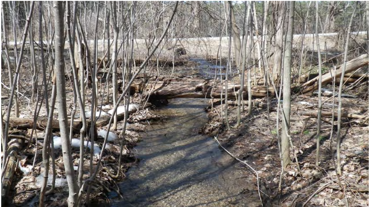
Photo 17: View looking upstream towards culvert outlet.
