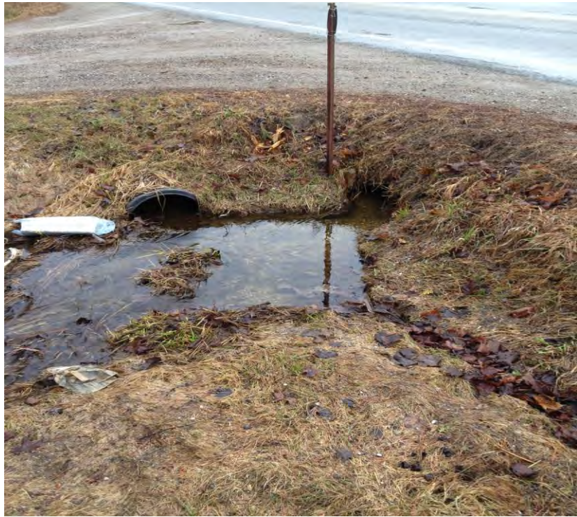
Photo 9: View looking upstream at culvert outlets.
