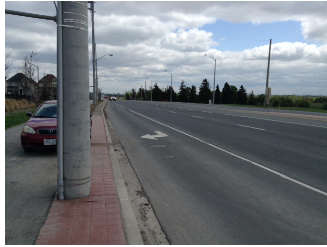
South Leg Mississauga Road
