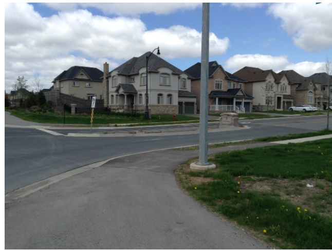
East Leg Beacon Hill Drive
