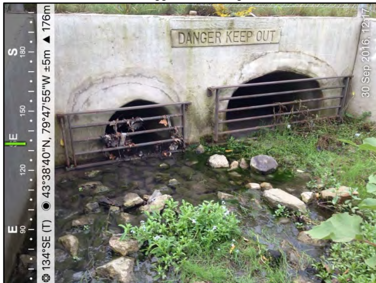
Photo 23: Outlet on right bank.
