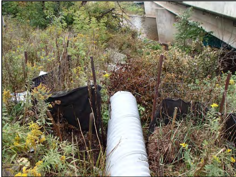
Photo 9: Outlet at top of bank on southeast side of bridge.
