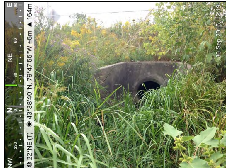
Photo 24: Outlet on right bank.
