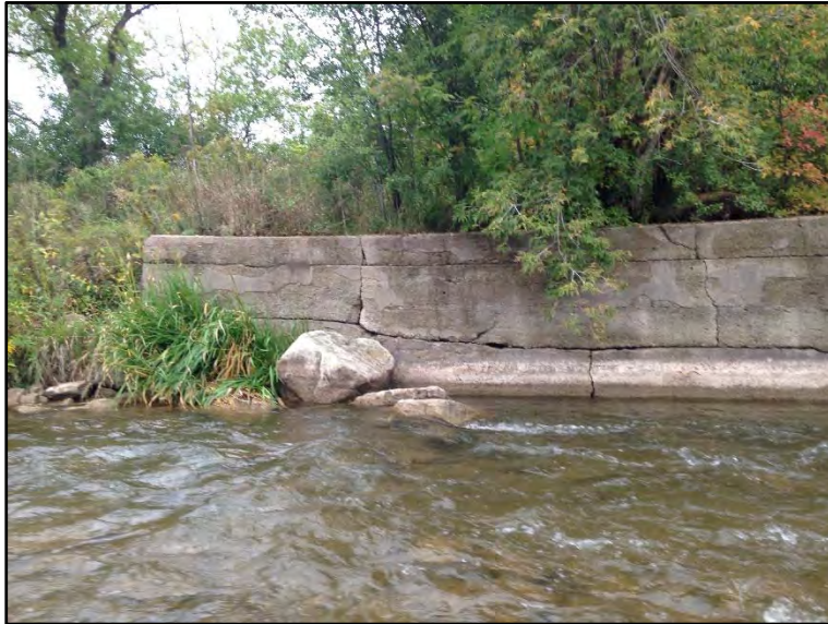
Photo 13: Concrete wall along left bank at downstream riffle.
