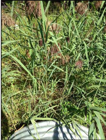
Photo 5: Looking down at outlet.
