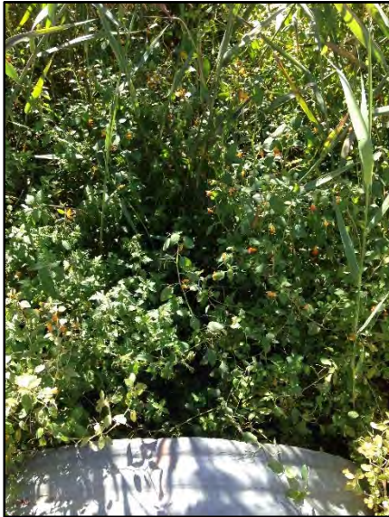
Photo 1: Looking down at inlet.
