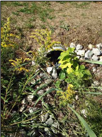
Photo 7: Placed riprap at outlet.
