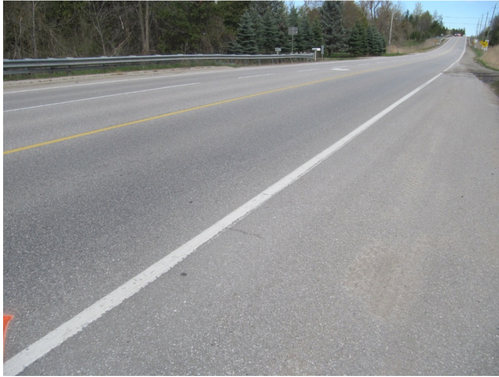
Photo 1: Pavement in good condition on North leg of intersection
