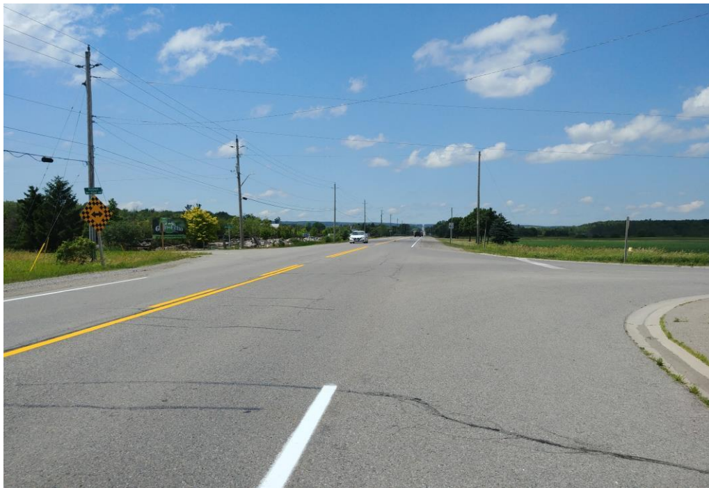
Photo 6: Airport Road at Sta. 12+900, Looking North
