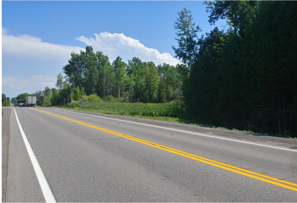
Photo 15: Airport Road at Sta. 17+150, Looking South
