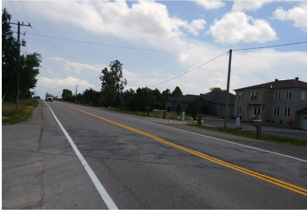
Photo 7: Airport Road at Sta. 13+880, Looking South
