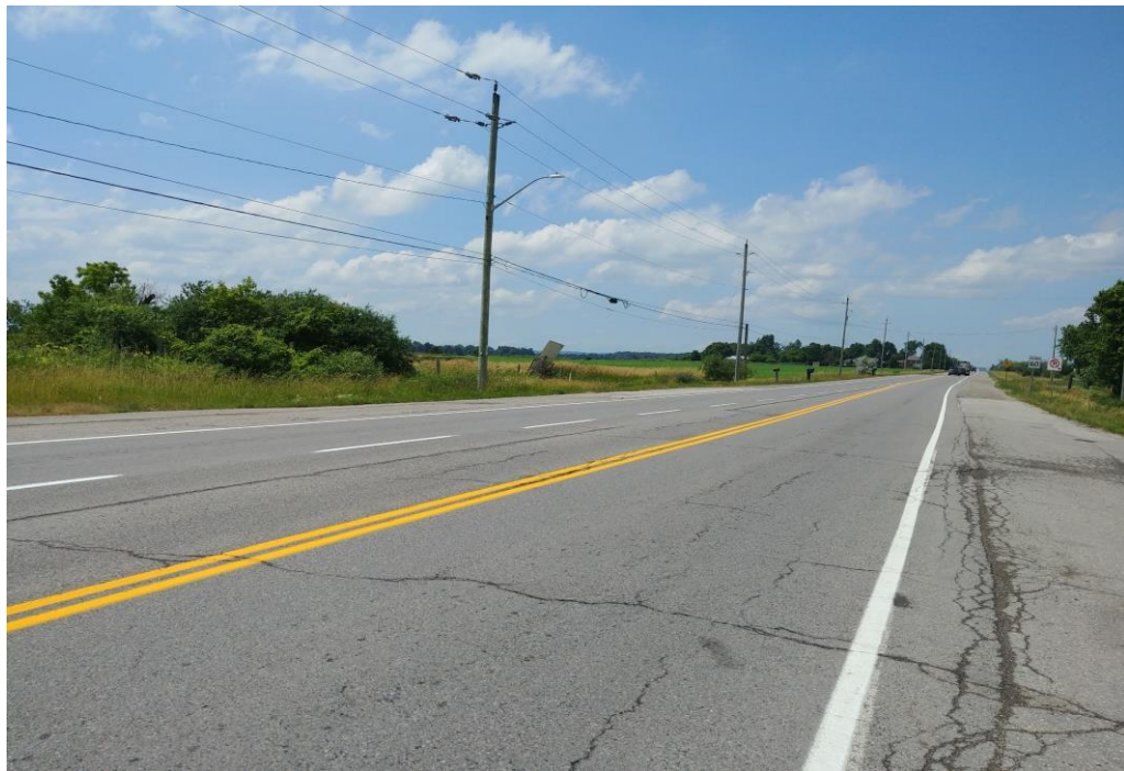
Photo 2: Airport Road at Sta. 9+900, Looking North
