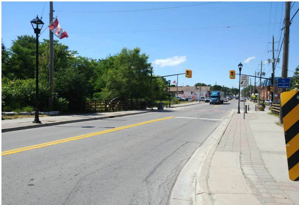
Photo 12: Airport Road at Sta. 15+720, Looking North
