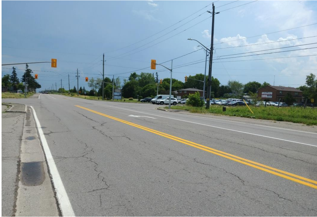
Photo 1: Airport Road at Sta. 9+900, Looking South at South Project Limit
