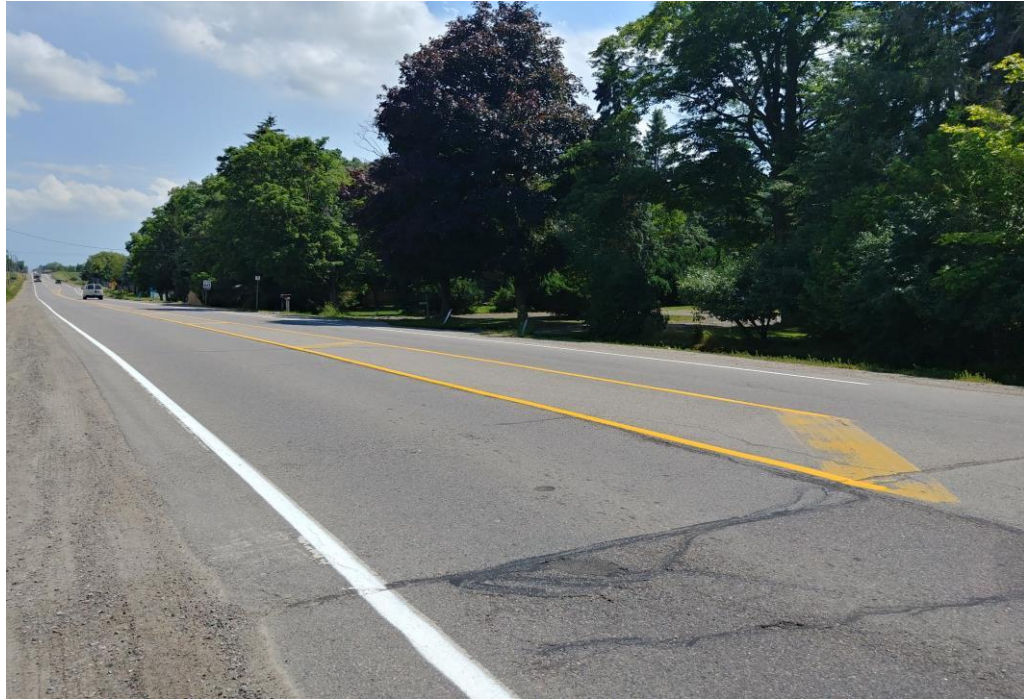
Photo 9: Airport Road at Sta. 15+200, Looking South
