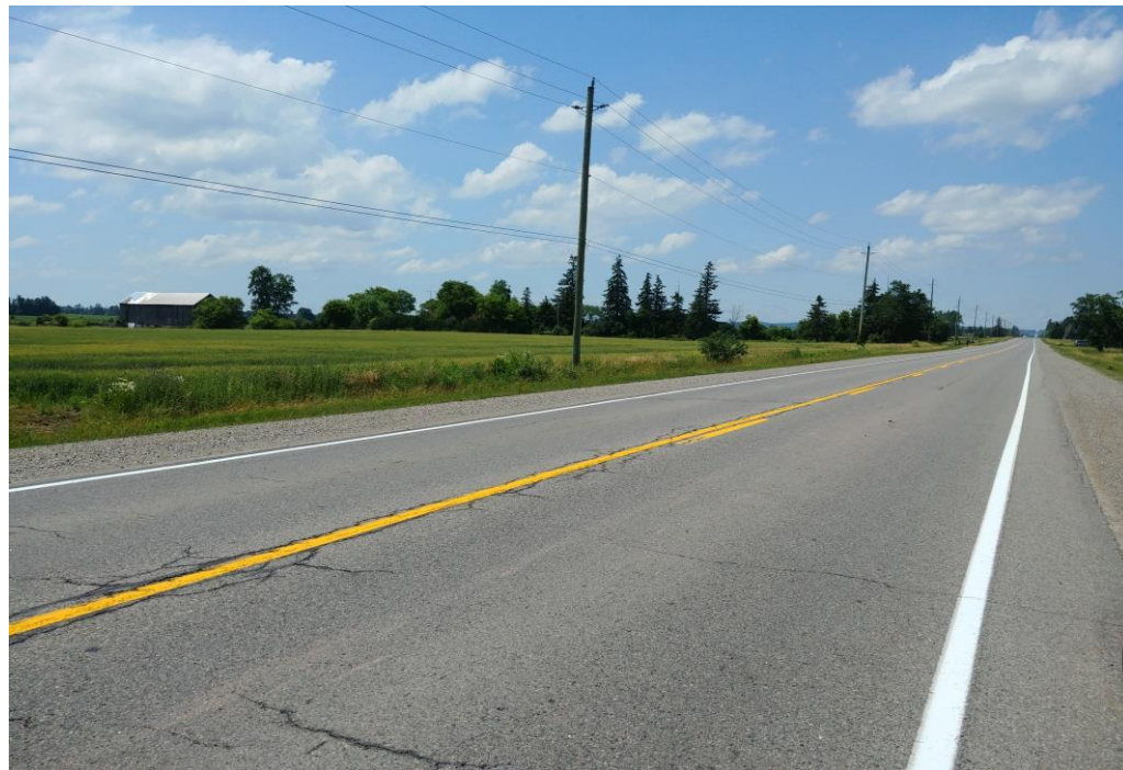
Photo 4: Airport Road at Sta. 11+100, Looking North
