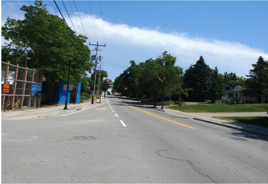
Photo 11: Airport Road at Sta. 15+720, Looking South
