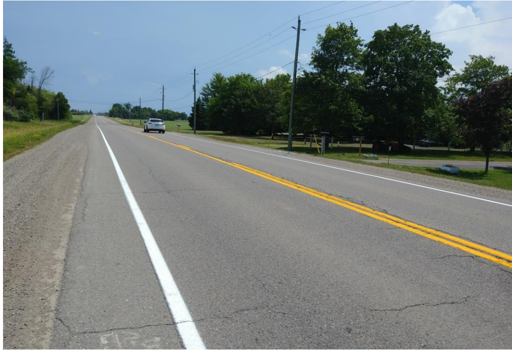
Photo 3: Airport Road at Sta. 11+100, Looking South
