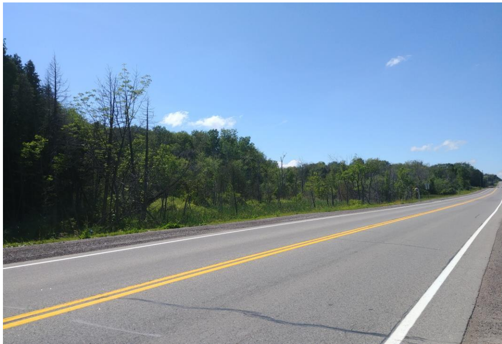
Photo 16: Airport Road at Sta. 17+150, Looking North at North Project Limit
