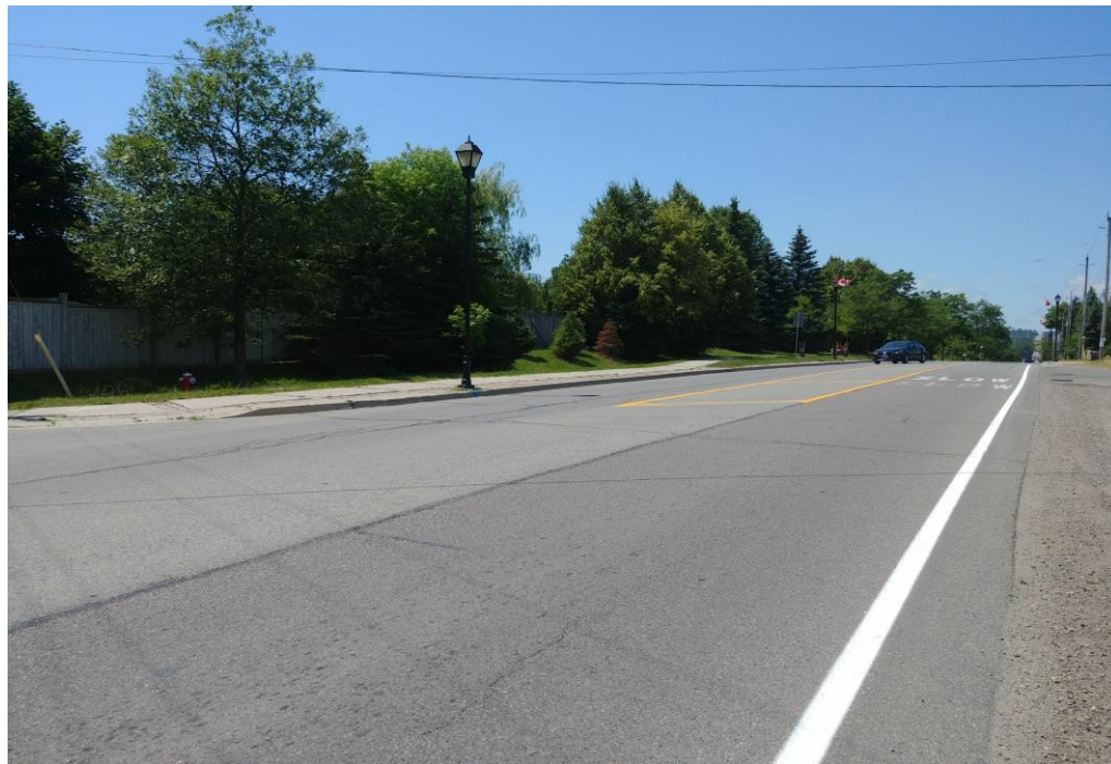
Photo 10: Airport Road at Sta. 15+200, Looking North
