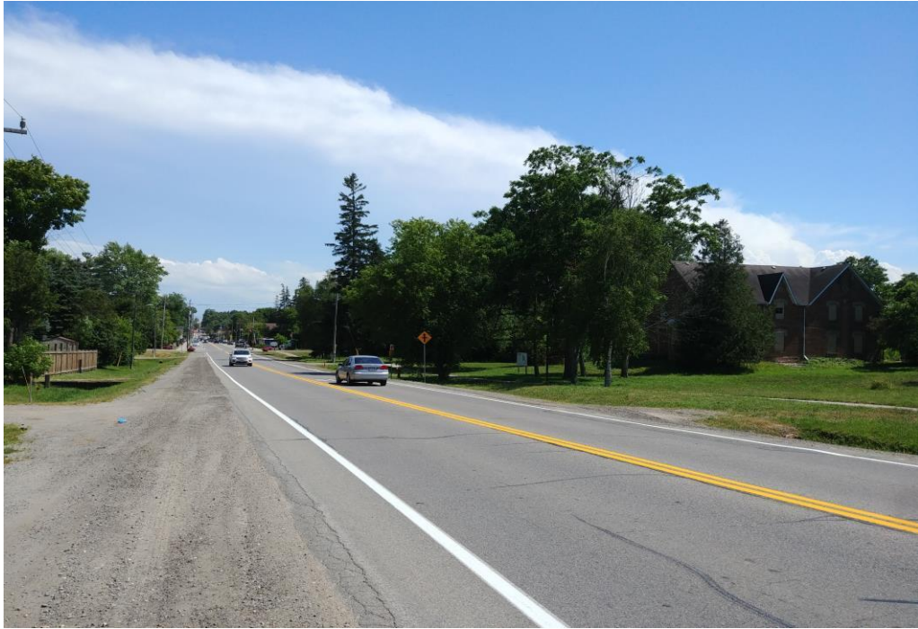
Photo 13: Airport Road at Sta. 16+440, Looking South
