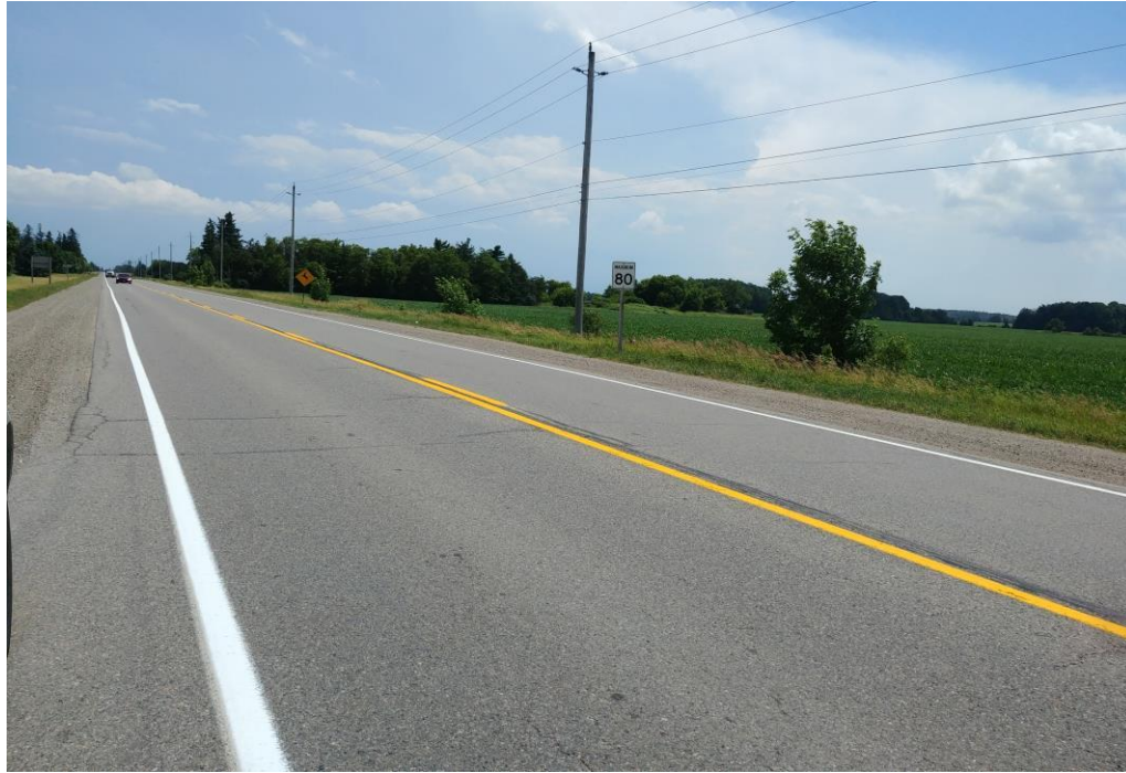
Photo 5: Airport Road at Sta. 12+900, Looking South
