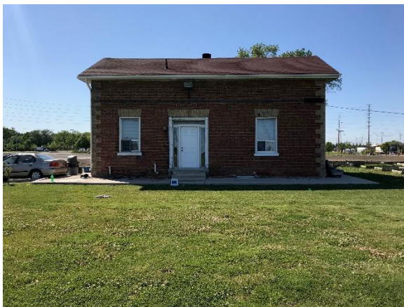
South elevation of the residence at 1411 Derry Road East.
