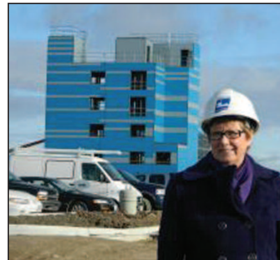
Pat stands in front of the new smoke tower at the Garry Morden Centre. The new fire training facility opens in spring 2012.
