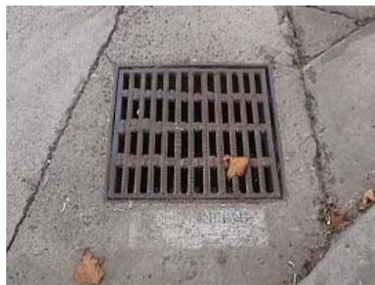
Figure 21: Catch Basin Grate
