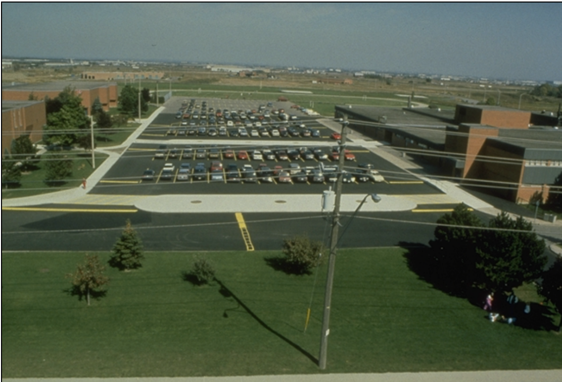
Photo 16: This photo is an example of a property designed to effectively deal with the movement of people onto and through the property. Section 5.1 School Grounds.
