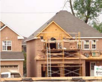
Construction Site in Brampton
