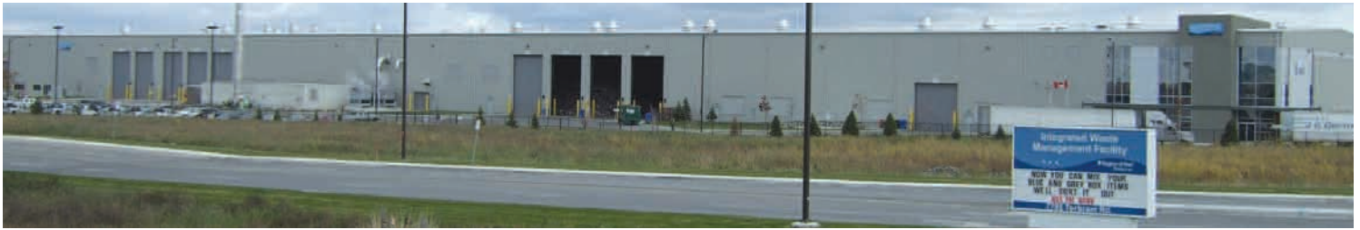
Peel Integrated Waste Management Facility
