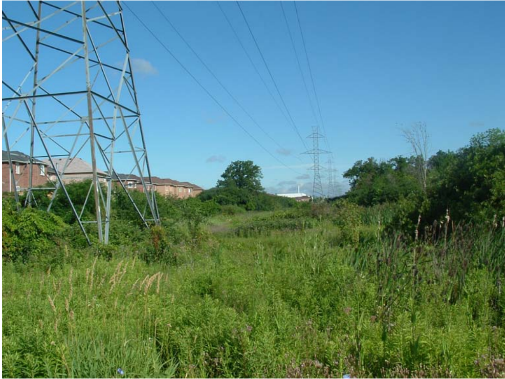
11. Parkway Belt West Corridor north of Eglinton Avenue East
