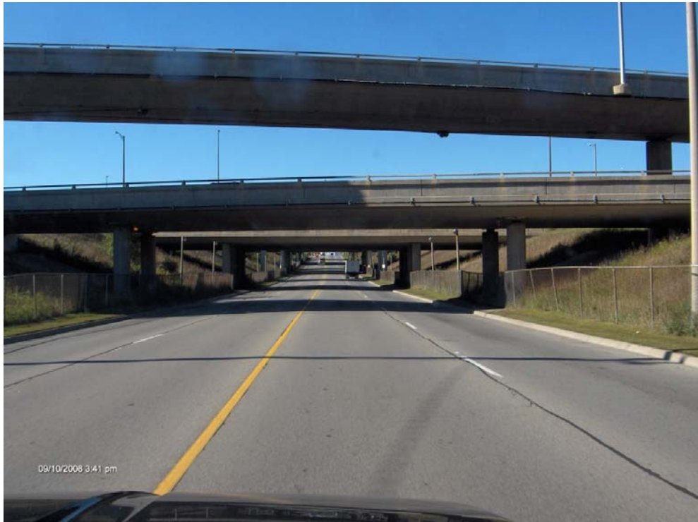
1. Tomken Road under Highway 401
