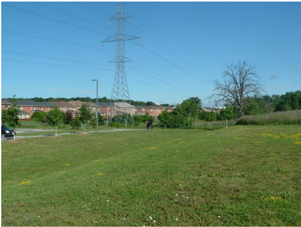
10. Parkway Belt West Corridor north of Eglinton Avenue East
