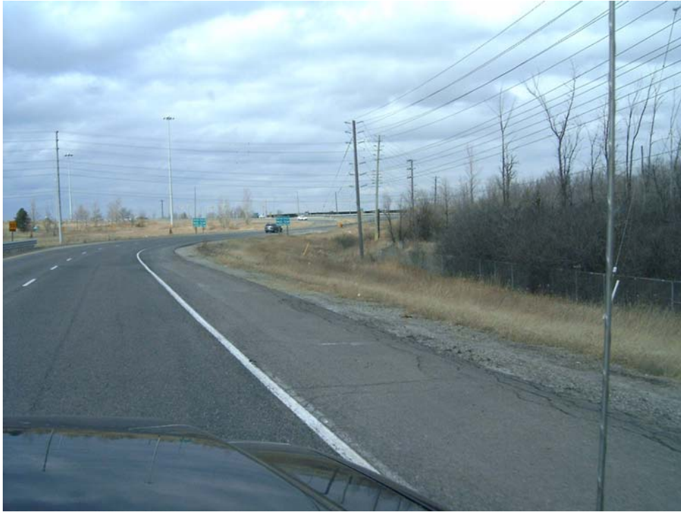
5. Eglinton Avenue East at Highway 403 Interchange
