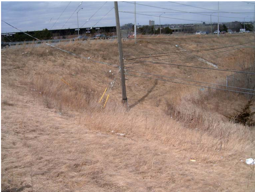
6. Eglinton Avenue East at Highway 403 Interchange
