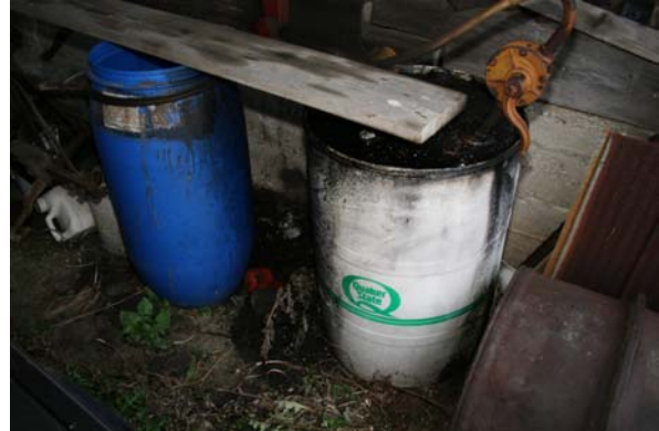
Photograph No. 8 Waste oil storage in Building D. Minor ground staining around drums.
