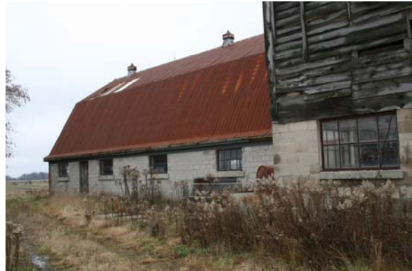
Photograph No. 2 View of Building B on Site.
