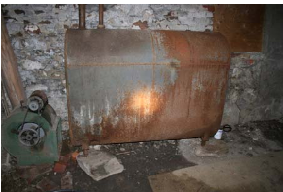
Photograph No. 11 AST in basement of Building A.
