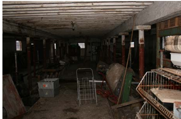
Photograph No. 4 Main level in Building B.
