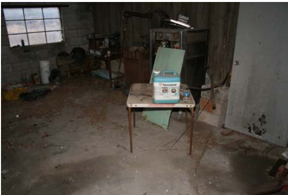
Photograph No. 9 Inside northwest portion of Building D.
