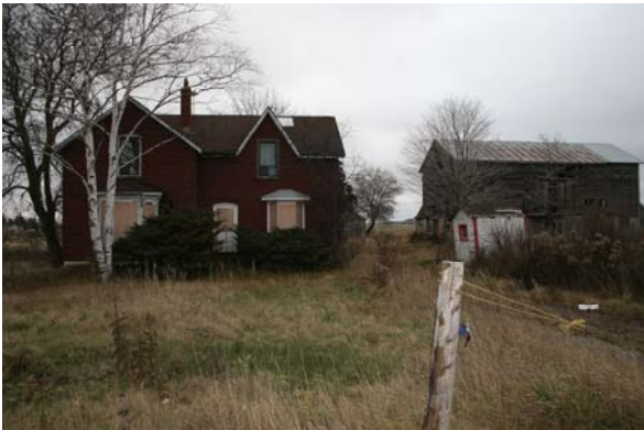
Photograph No. 3 Building A and B on Site.
