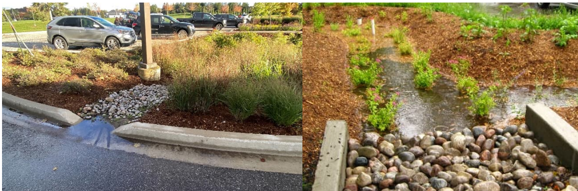
Figure 6.5 – SWM Alternative 4 Bioretention Facilities
