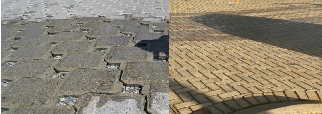
Figure 6.6 – SWM Alternative 5 Permeable Pavement
