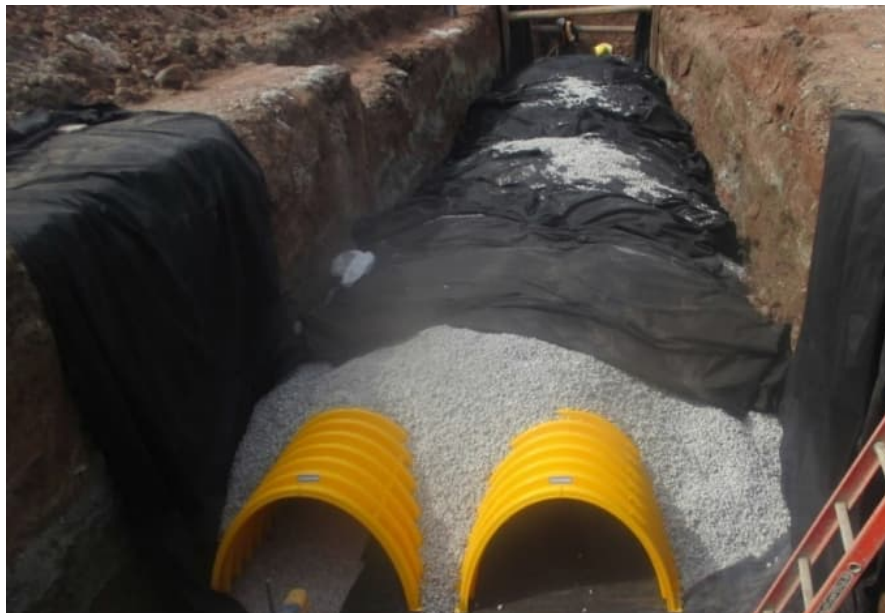
Figure 6.8 – SWM Alternative 7 Superpipe Storage
