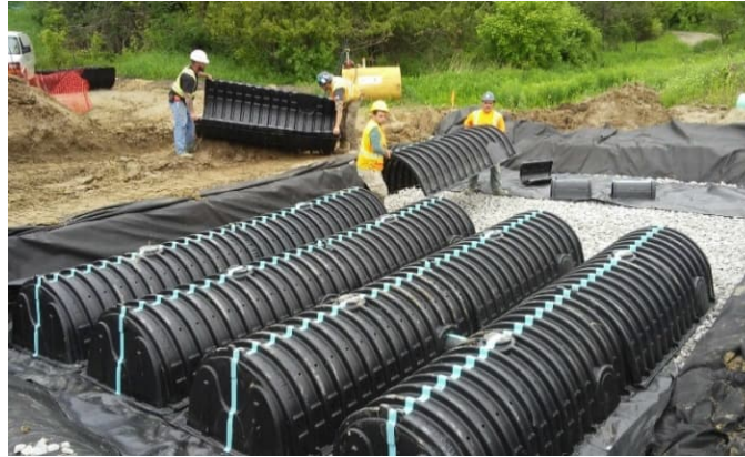
Figure 6.9 – SWM Alternative 8 Infiltration Trenches
