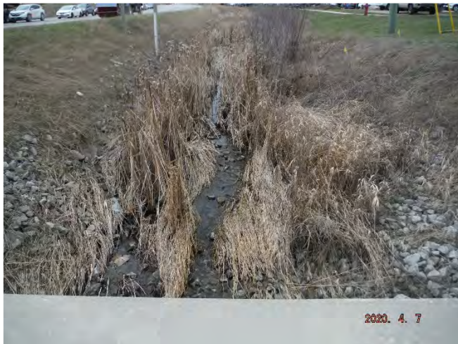
Robinson Creek northeast of RR50 and Mayfield Road looking north along east side of RR50 (April 7, 2020).
