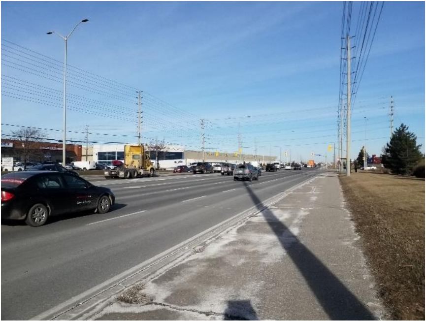
Plate 6: Derry Road East, looking northeast towards Bramalea Road.
