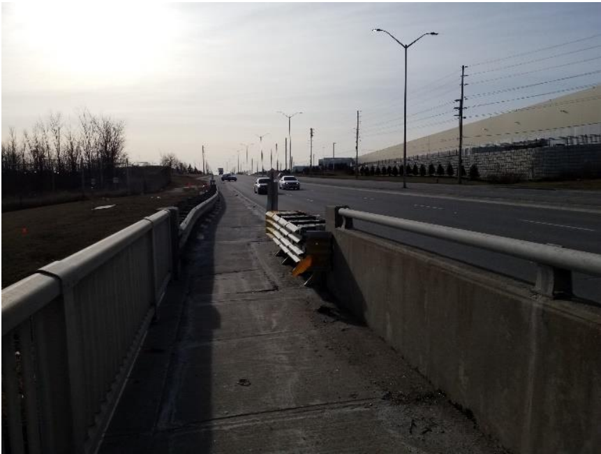
Plate 8: Derry Road East, looking southwest towards Bramalea Road.
