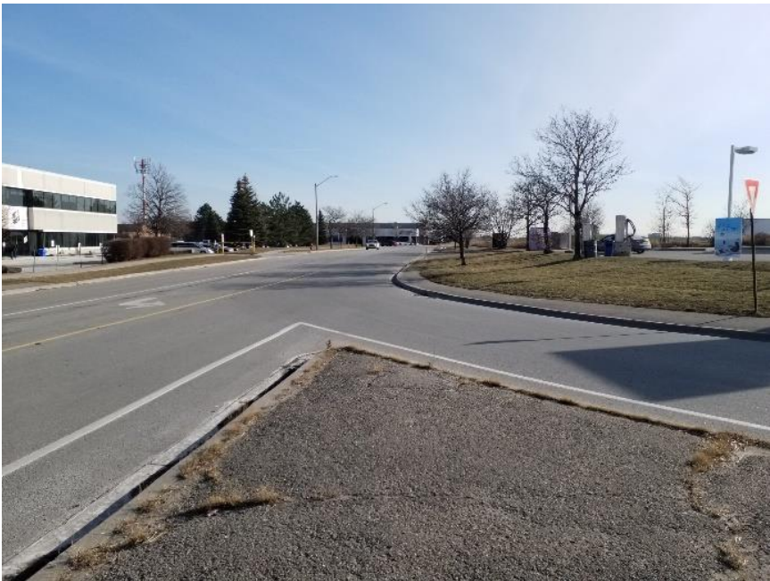
Plate 3: Menkes Drive, looking southeast.
