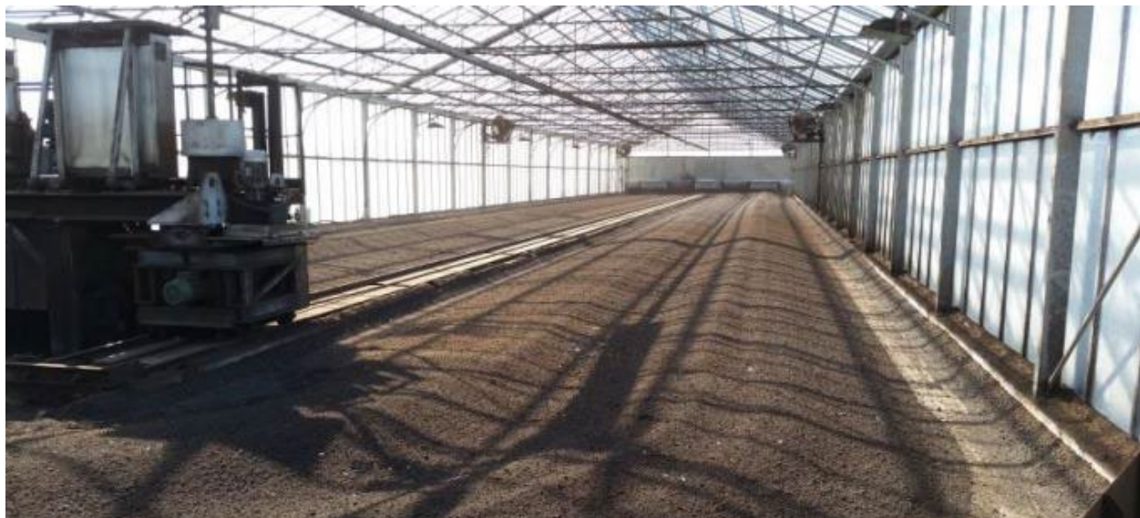
Figure 3-11 A Solar Drying Facility
