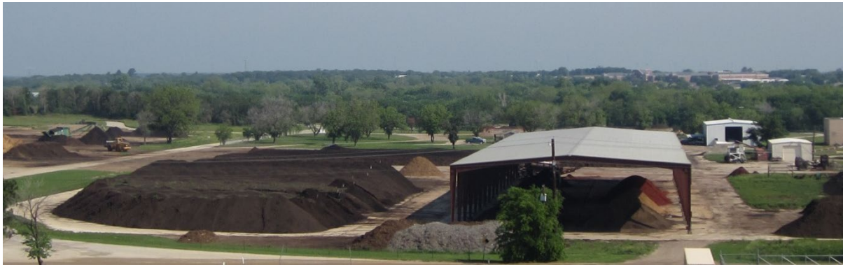
Figure 3-15 Denton, Aerated Static Pile, Composting Facility at Columbus, OH
