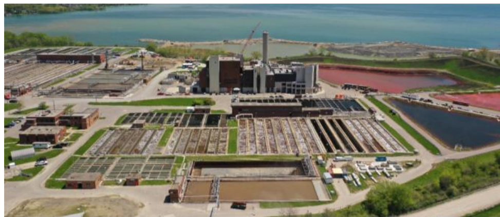
G.E. Booth Wastewater Treatment Plant (518 MLD)
