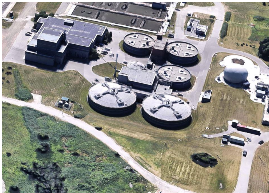
Anaerobic Digesters, Clarkson WWTP
