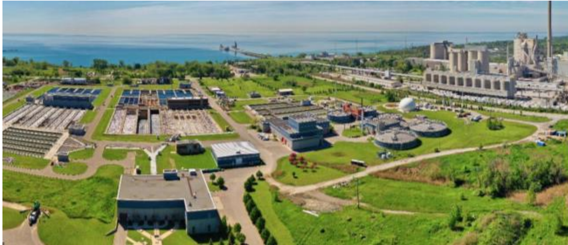
Clarkson Wastewater Treatment Plant (350 MLD)
