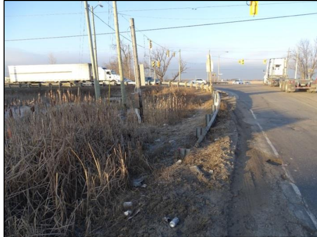
Figure 12: Turned Down Approach Treatment Colerain Drive and Region Road 50
