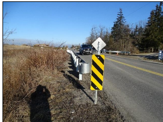
Figure 21: Steel Guide Rail Leaving-End (Clarkway Drive and Countryside Drive)
