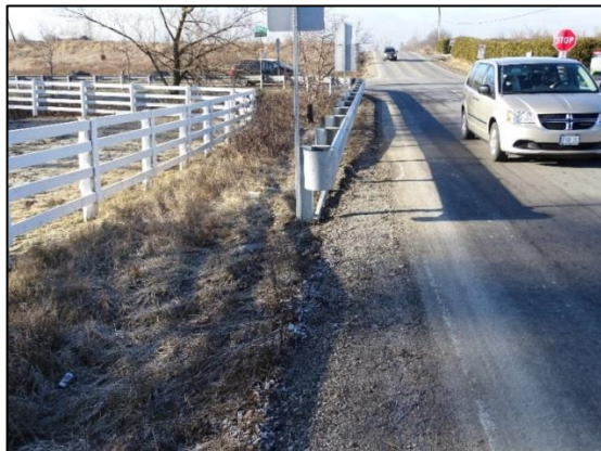
Figure 21: Steel Guide Rail Leaving-End (Clarkway Drive and Countryside Drive)
