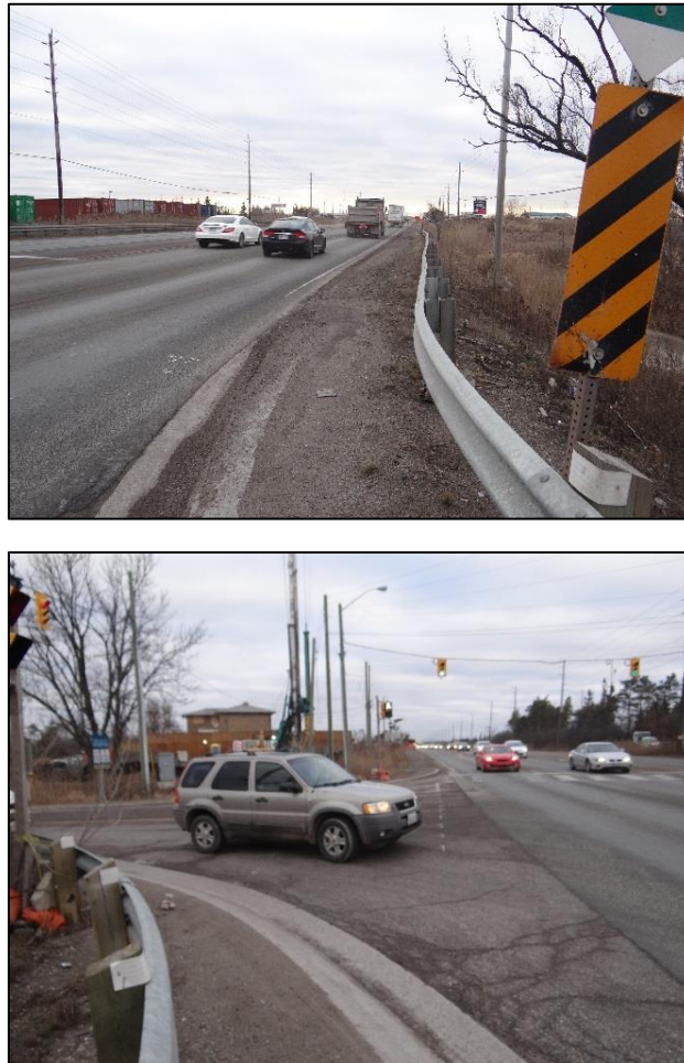
Figure 11: Pedestrian Sidewalks (Coleraine Drive and Regional Road 50)
