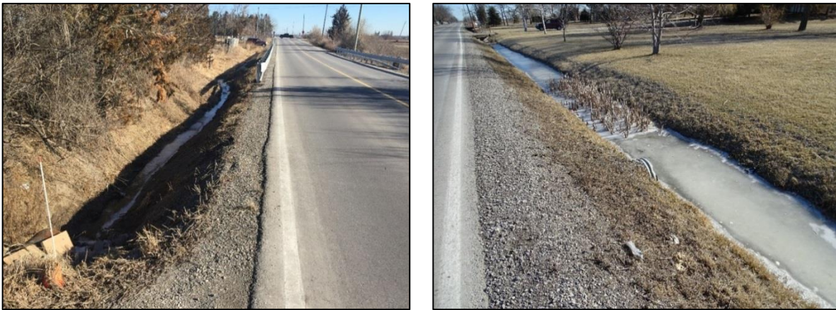
Figure 26: Side Slopes along Countryside Drive
