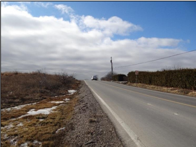
Figure 15: Narrow Shoulders along the Clarkway Drive Corridor
