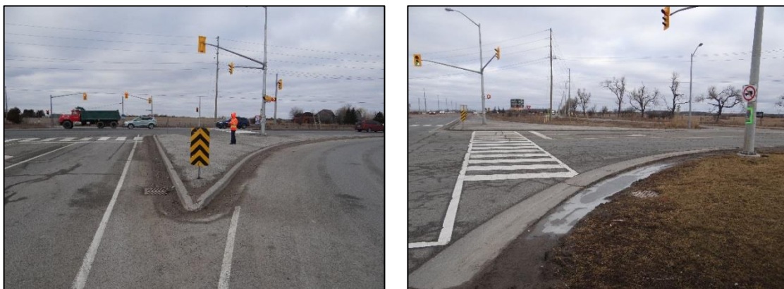
Figure 31: Lack of Pedestrian Infrastructure (Countryside Drive and Regional Road 50)
