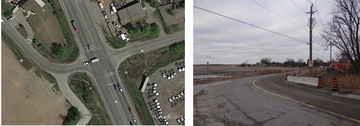
Figure 3: Skewed Intersection (Colerain Drive and Region Road 50)
