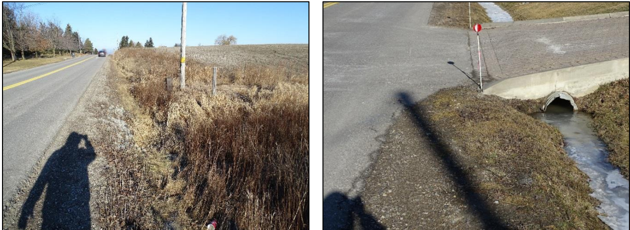
Figure 17: Fixed Objects along the Clarkway Drive Corridor
