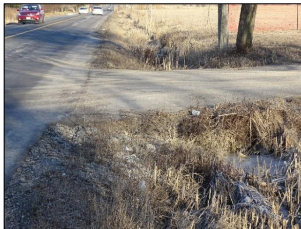
Figure 6: Narrow Shoulders along the Coleraine Drive Corridor
