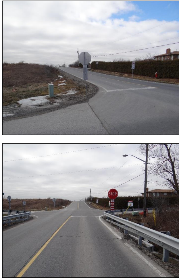
Figure 13: Intersection at Clarkway Drive and Countryside Drive
