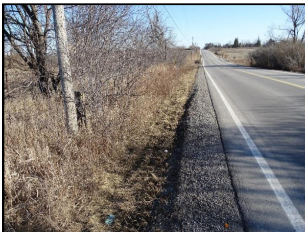
Figure 25: Narrow Shoulders along Countryside Drive
