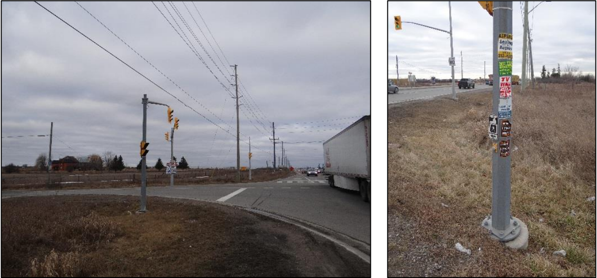
Figure 30: Accessibility of Pedestrian Push Button (Countryside Drive and Regional Road)
