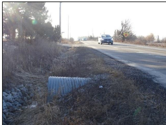
Figure 7: Side Slopes along the Coleraine Drive Corridor
