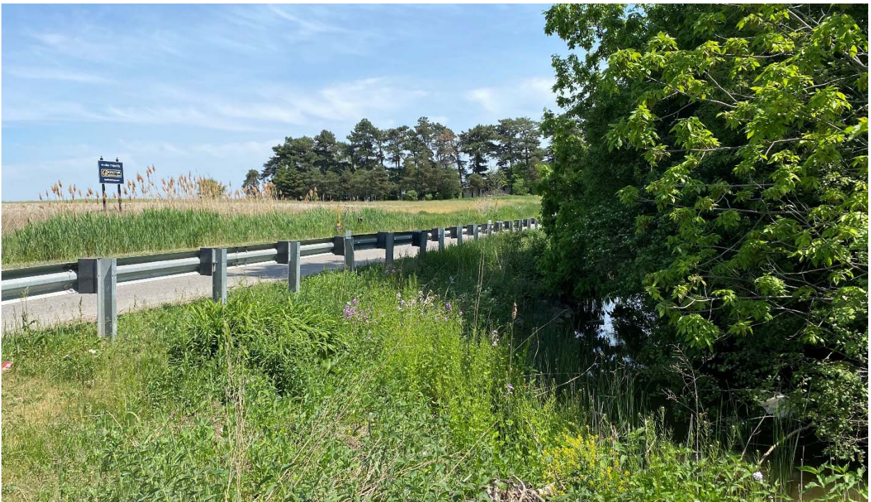
Image 11: Looking south on the east side of Clarkway Drive. – The reflection of Clarkway Tributary can be seen beneath the shadows of overhanging trees. From this point south 400 metres the tributary clings to the roadside necessitating steel guardrails. It is assumed significant channel protection, alignment, and restoration will be needed for the proposed corridor improvements to take place.
