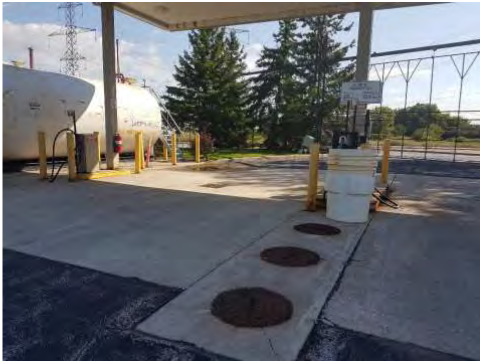
Plate 4: 7405 E Danbro Cres (Penske Truck Rental), Underground Storage Tank (USTs), located at the east end of the property.
