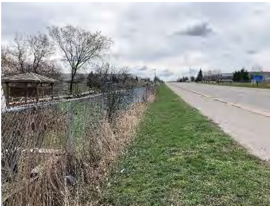
Plate 6: Meadowvale Boulevard, looking southeast. Visible on the left of the photo is recreational space (dog park) and on the right, the Meadowvale North Pumping Station.
