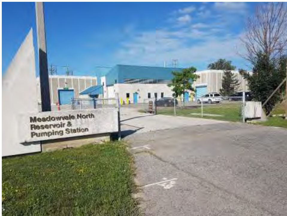
Plate 7: Meadowvale North Reservoir & Pumping Station at 2720 Meadowvale Blvd.
