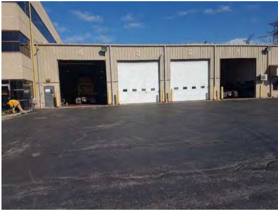
Plate 6: 7405 E Danbro Cres (Penske Truck Rental), truck maintenance facility located at the west end of the property.
