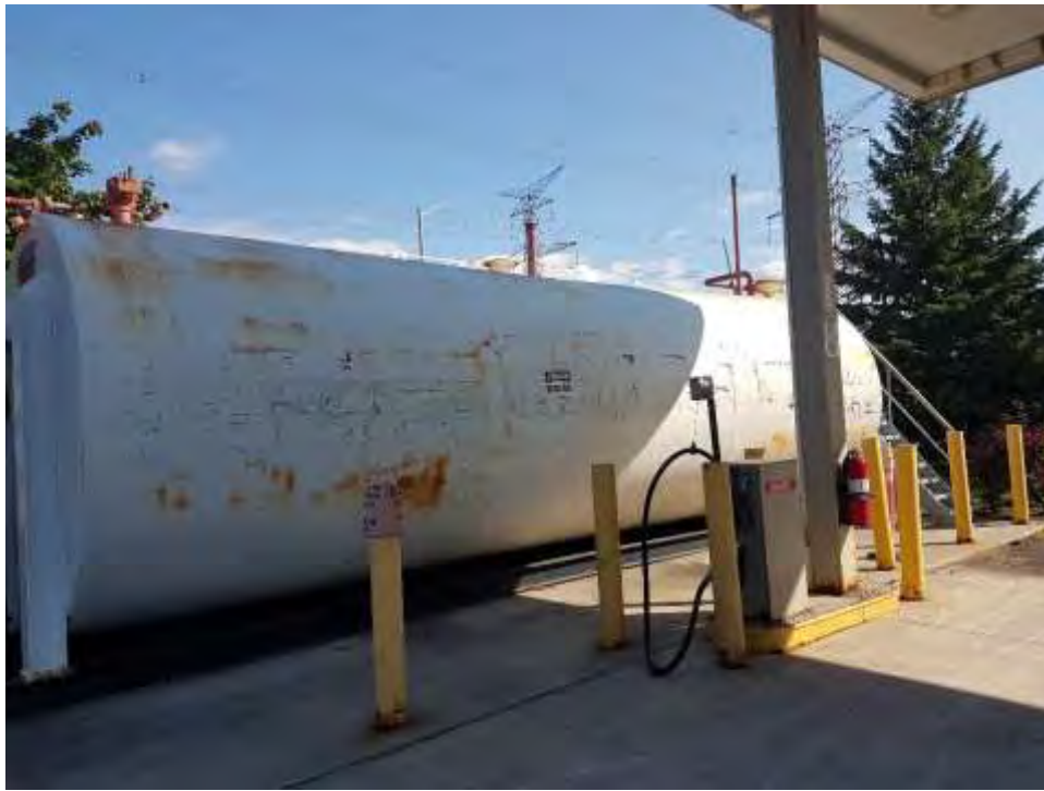
Plate 3: 7405 E Danbro Cres (Penske Truck Rental), Aboveground Storage Tank (AST), located at the east end of the property.
