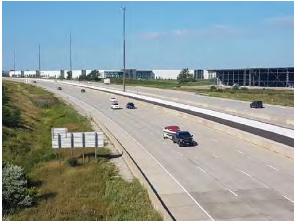
Plate 9: Highway 407, looking west from the Heritage Road bridge.
