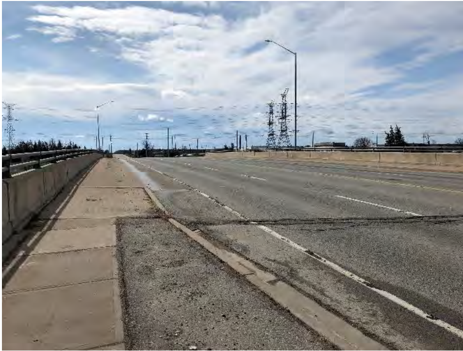
Plate 3: View south along the bridge carrying Heritage Road over Highway 407.
