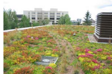
Living 'Green' Roof
