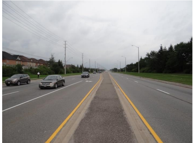
Plate 2: Airport Rd. with center median, looking north from Braydon Blvd/Stonecrest Dr.
