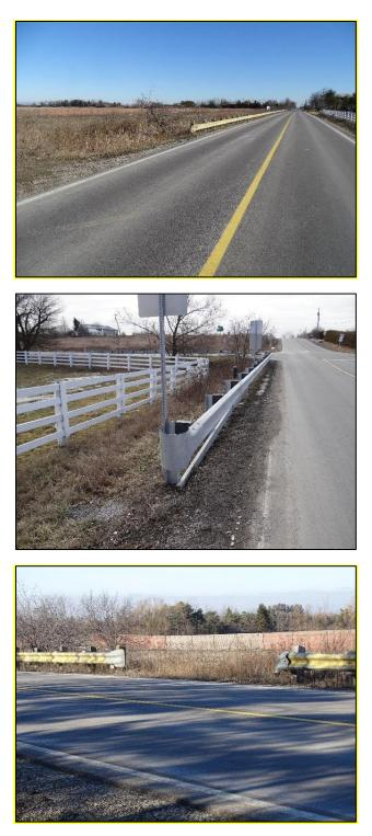
Figure 34: Steel Guide Rail Leaving-End along Countryside Drive
