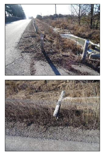
Figure 20: Damaged Cable Guide Rail along the Clarkway Drive
