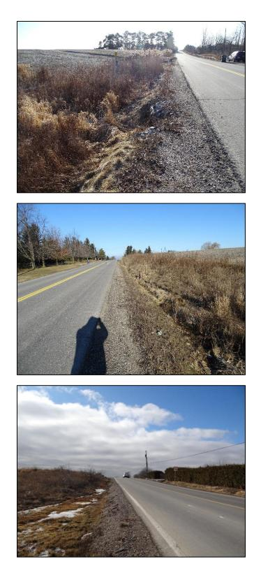
Figure 15: Narrow Shoulders along the Clarkway Drive Corridor
