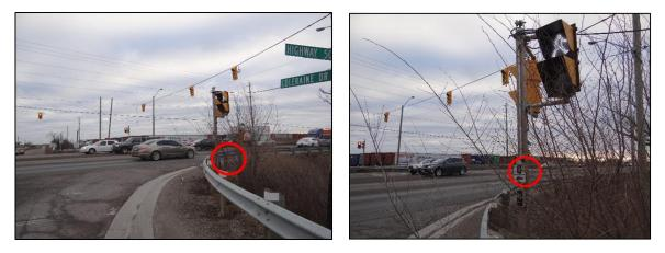
Figure 10: Obstructed Pedestrian Push Button (Colerain Drive and Regional Road 50)
