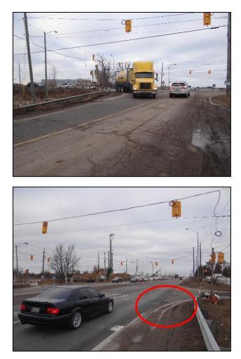
Figure 2: Limited Turning Radius (Coleraine Drive and Region Road 50)
