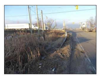
Figure 12: Turned Down Approach Treatment Colerain Drive and Region Road 50
