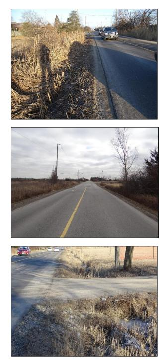
Figure 6: Narrow Shoulders along the Coleraine Drive Corridor
