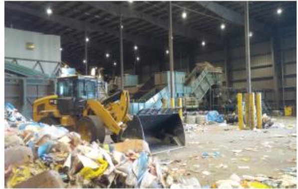
After: Combination of 200W and 100W integrated LED light fixtures. Illumination is 10 times brighter!
